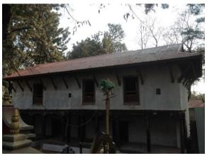
The Sattal is restored over its original foundation and used almost artistic wooden material of original structure. The ground floor of the Sattal was occupied illegally and also partitioned for residential purpose. After the restoration of the Sattal, it is reopened the Dalan for cultural activities. Replacing the mud mortar the Sattal is restored using Lime mortar. All the responsibility of restoration was taken by PADT.
