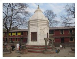
restoration work; but all the wood are replaced by new and the mud mortar is replaced by Lime mortar.
