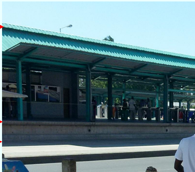
Photo 31: Example of BRT Platform with raised floor for exclusive use of BRT passengers (DAR)
