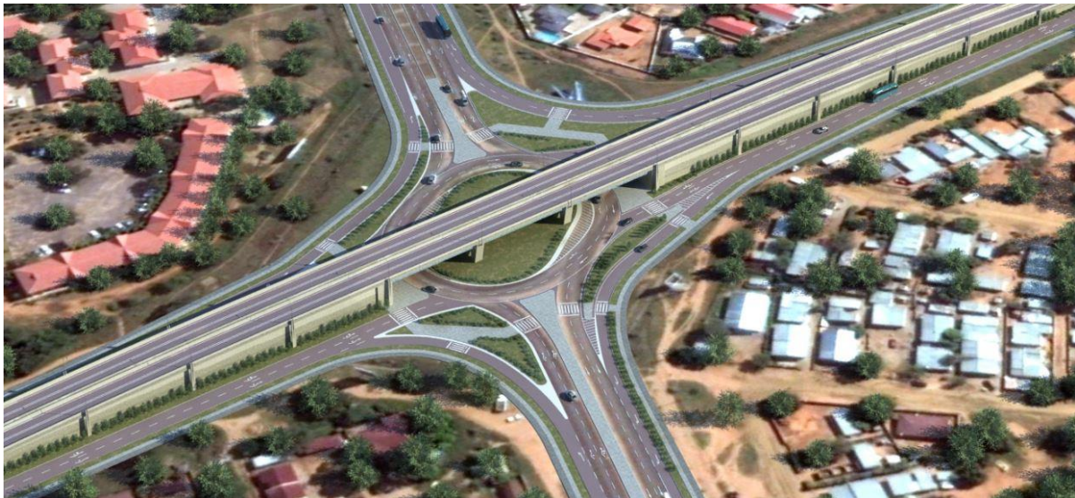
Figure 18: Visual image of diamond type interchange with roundabout at the ground level and provision for NMT facilities
