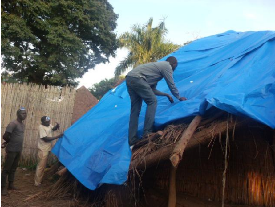
Completion of fixing the internal weather proof layer.
