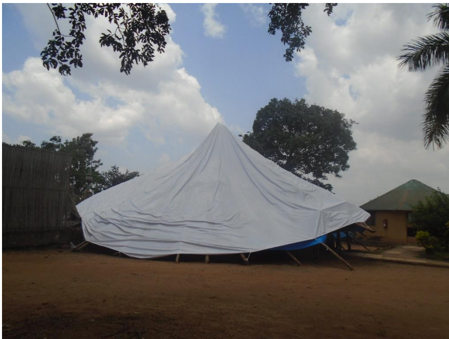
Fixation of the external weather proof layer.
