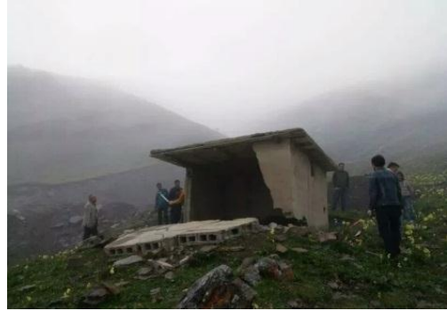
Figure 1: Tianwo coal mining—demolishing facilities on the ground
