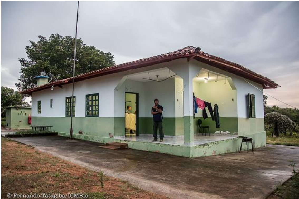
Figure 4: Headquarters of the Chapada de Nova Roma Ecological Station, with the constant presence of public servers from SECIMA-GO, ensuring the protection of the area.
