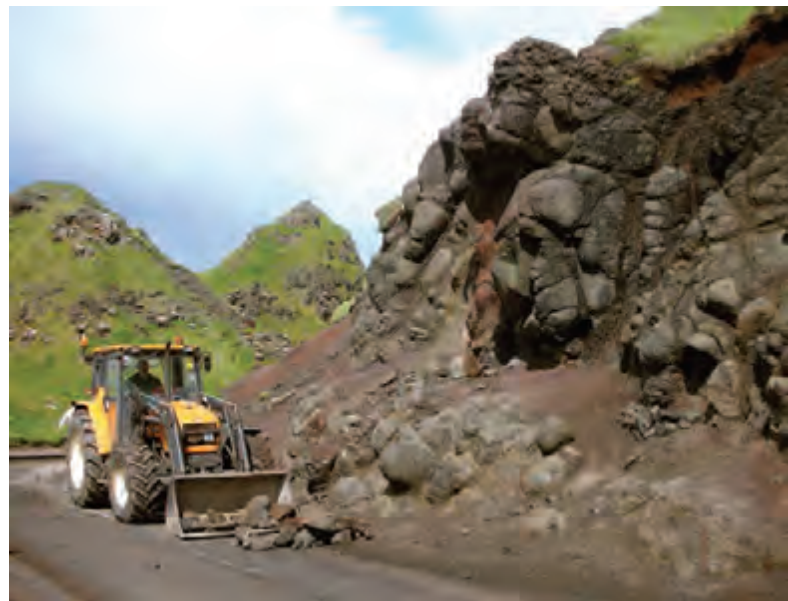
National Trust clearing debris from a recent slope failure (photo provided by National Trust)
