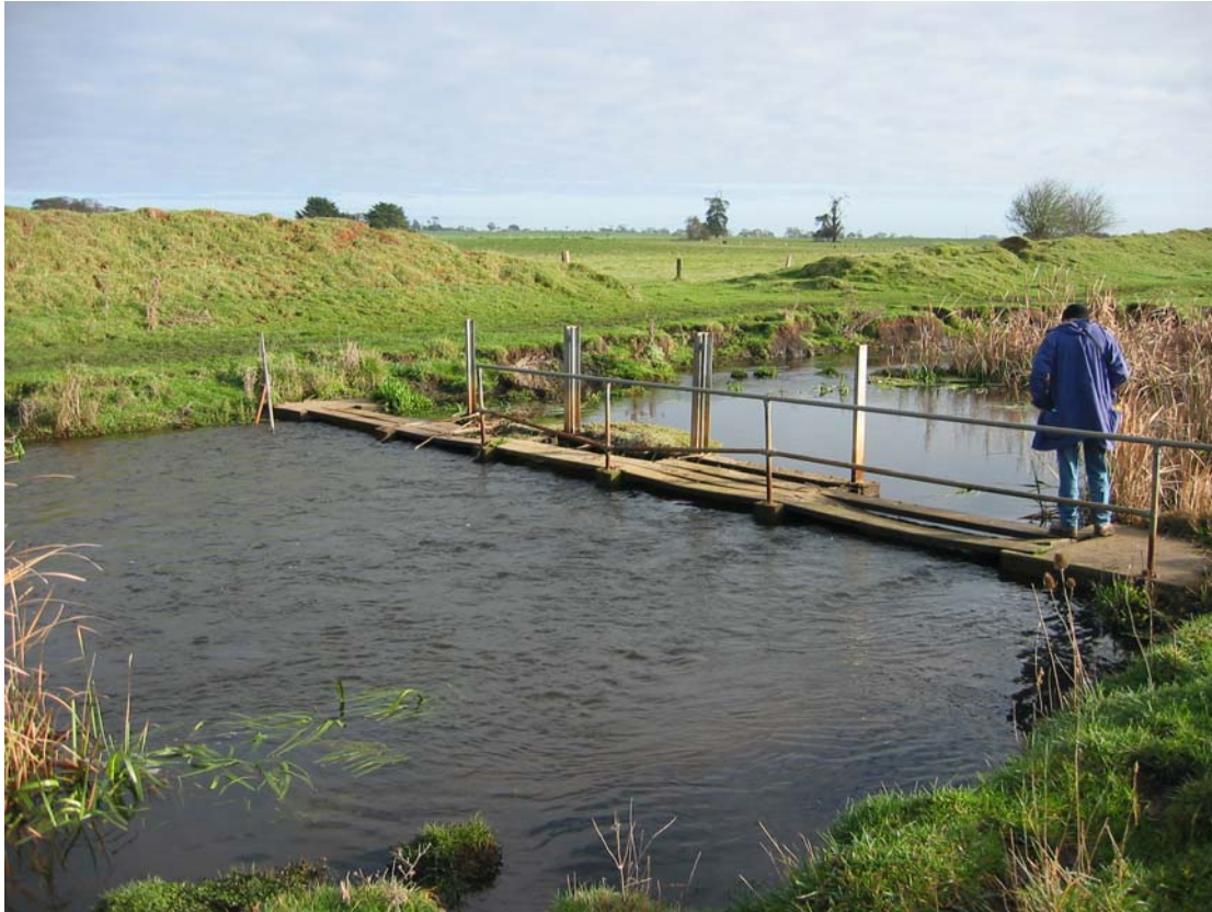
Figure 31. Weir constructed at the northern end of Lake Condah, some time in 1990, in order to divert flows from Condah Drain into Lake Condah. Flow is right to left. Photo: C. Gippel, 19/07/2006.
