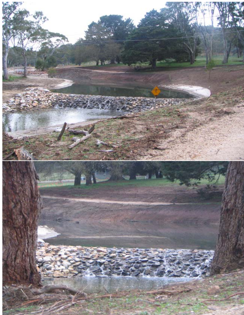
Figure 126. Example of grouted rock weir structure. Note that detail of the illustrated structure differs from that of the structure proposed for Lake Condah. Photo credit: Geoff Fisher (Australian Water Environments).
