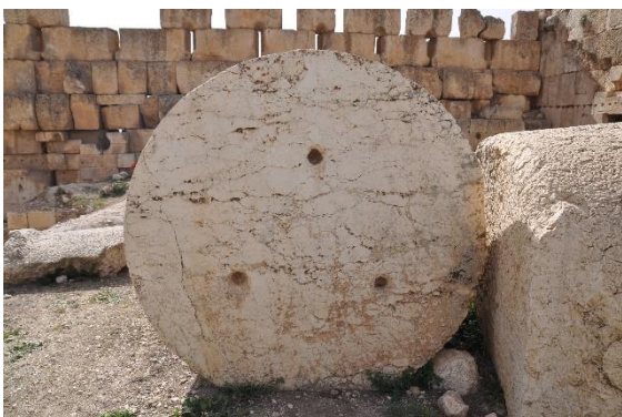
Figure 26 – View of one of the ends of one of the fallen column shaft stones. The three drilled holes would have received metallic anchors to secure one stone top of the other. The metallic anchors would have been set in molten lead.
