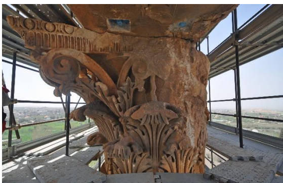
Figure 31 – One of the Corinthian capitals as seen looking westward. Carving is highly ornate but is only present on the south side of the Capital.
