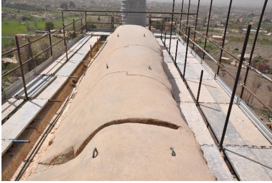
Figure 38 – View of the concrete cap looking eastward. The concrete is smooth and rounded in order to shed water to the original guttering system on the south and off of the stone lintel on the north.
