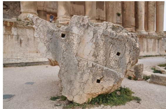
Figure 37 – Side view of the frieze unit showing the tothing of one stone to the other. Small square holes either used to receive metal towels, to hoist the stone into place, or both.
