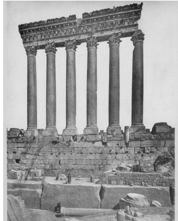
Figure 7 – View of the Jupiter Colonnade as seen from the south. Characteristic damage of the frieze in the middle of the stone lintel can be seen. The eastern portion of the stone lintel (right) extends no further than the centerline of the column. Photograph taken during the German mission, circa 1900.
