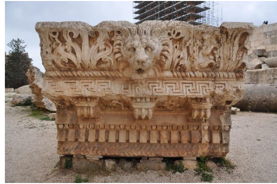
Figure 36 – A unit of the frieze that has fallen to the ground. Note the high degree of ornamental carving, much of which was put in place after the stone was set atop the Colonnade.
