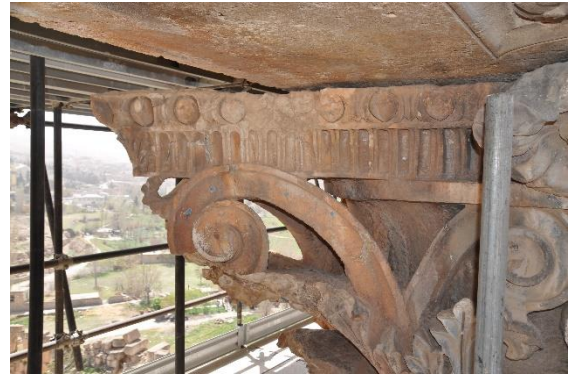
Figure 32 – Close up view of one of the Corinthian capital scrolls revealing its delicate nature and deep carving. Metallic anchors added by the French Mission can easily be seen because they have been painted with blue paint.
