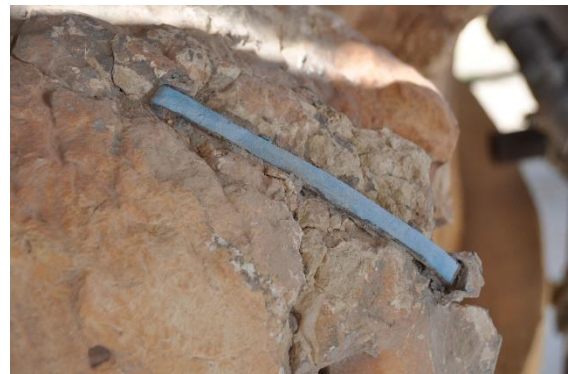
Figure 33 – Close up view of metallic anchor which appears to be wrought iron and square in profile, and not the carbon steel and circular in profile of which the French Mission anchors are composed. This anchor is believed to be from the Roman era and installed as a repair during the initial construction of the temple.
