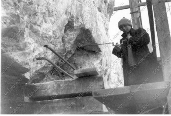
Figure 15 – Holes to receive ferrous metal rods in the stone lintel are being drilled by hand. Photograph taken during the French Mission, circa 1930s.
