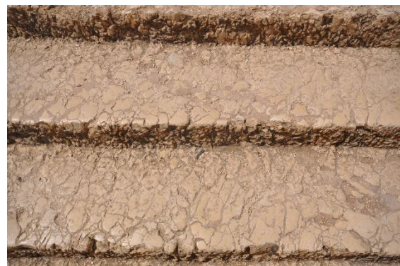
Figure 24 – Disaggregation of the limestone as seen on the steps leading up to the temple of Bacchus.
