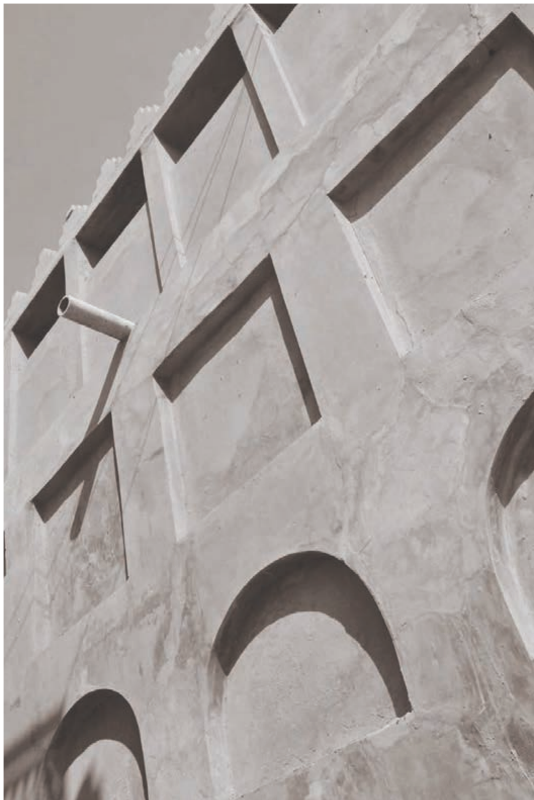
Sequence of niches and buwwādgīr on Murad House exterior facade
