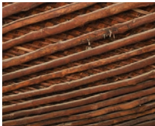
Traditional construction material: mangrove beam ceiling and unplastered coral stone wall
