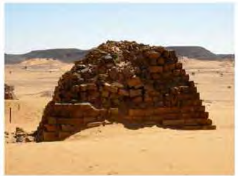
DSCN3767.JPG, Structural Deterioration of Pyramids, Northern Cemetery
