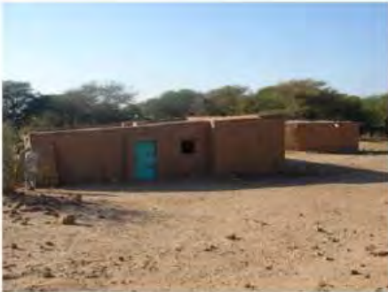
DSC06262.JPG, Redundant/Inappropriate Visitor Infrastructure, Royal City
