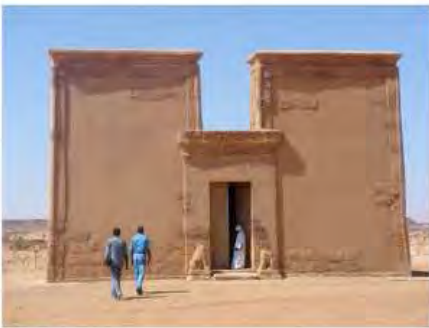
DSC06216.JPG, Musawwarat - Re-erected Lion Temple, Restoration Works
