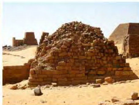
DSCN3778.JPG, Structural Deterioration of Pyramids, Northern Cemetery
