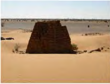
DSCN3854.JPG, Structural Deterioration of Pyramids, Southern Cemetery
