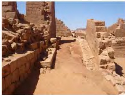
DSC06199.JPG, Musawwarat - Great Enclosure, Restoration Works
