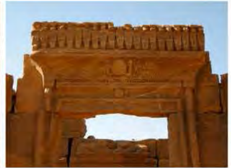
DSCN4016.JPG, The Kiosk - Naqaa, Naqaa, Structural Instability of Walls/Collapse of Archaeological Features
