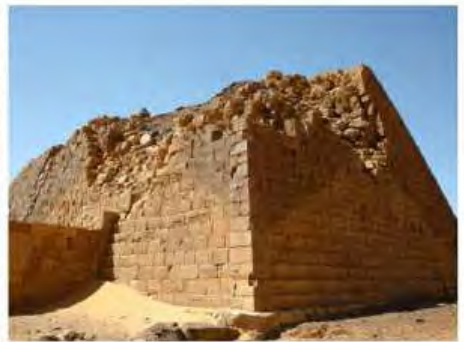
DSCN3764.JPG, Structural Deterioration of Pyramids, Northern Cemetery
