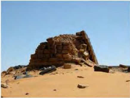
DSCN3795.JPG, Structural Deterioration of Pyramids, Southern Cemetery
