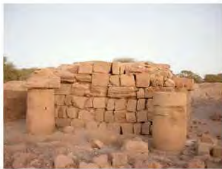
DSCN3987.JPG, Structural Instability of Walls/Collapse of Archaeological Features, Royal City
