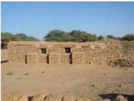
DSC06265.JPG, Redundant/Inappropriate Visitor Infrastructure, Royal City
