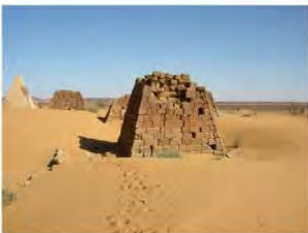
DSCN3864.JPG, Structural Deterioration of Pyramids, Southern Cemetery
