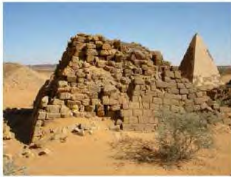
DSCN3843.JPG, Structural Deterioration of Pyramids, Southern Cemetery
