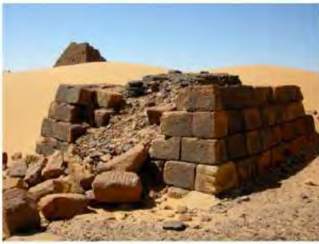
DSCN3804.JPG, Structural Deterioration of Pyramids, Southern Cemetery
