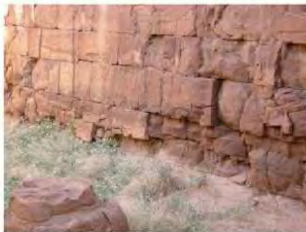
DSCN4027.JPG, Lion Temple B300 - Naqaa, Naqaa, Vegetation Damage, Degradation of Stone/Masonry Elements, Inappropriate/ Inexistent Site Drainage
