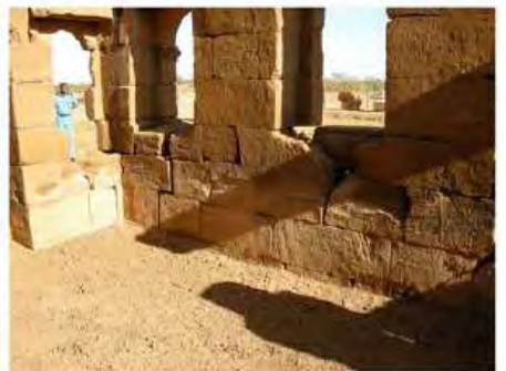
DSCN4008.JPG, The Kiosk - Naqaa, Naqaa, Degradation of Stone/ Masonry Elements, Inappropriate/Inexistent Site Drainage
