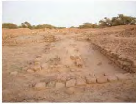
DSCN3966.JPG, Inappropriate Dumping of Excavation Spoils, Inappropriate/Inexistent Site Drainage, Structural Instability of Walls/ Collapse of Archaeological Features, Royal City
