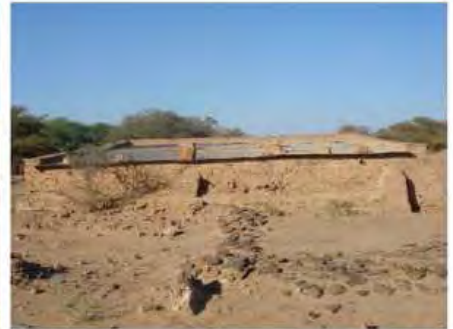
DSC06264.JPG, Redundant/Inappropriate Visitor Infrastructure, Royal City
