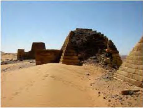
DSCN3747.JPG, Structural Deterioration of Pyramids, Northern Cemetery
