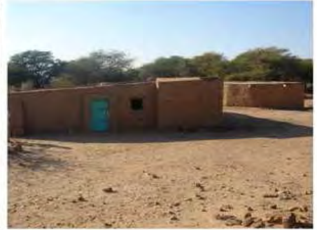
DSC06261.JPG, Redundant/Inappropriate Visitor Infrastructure, Royal City
