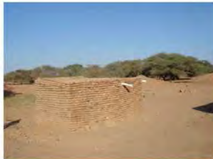
DSC06266.JPG, Redundant/Inappropriate Visitor Infrastructure, Royal City
