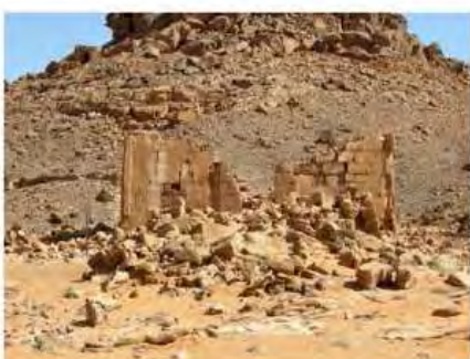
DSCN4139.JPG, Naqaa, Temple F, Structural Instability of Walls/Collapse of Archaeological Features, Structural Instability of Walls/Collapse of Archaeological Features
