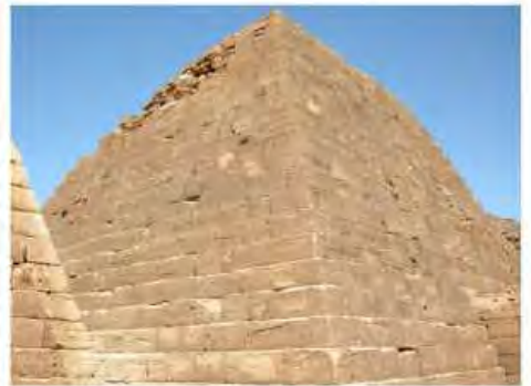
DSCN3755.JPG, Public Safety Hazard, Northern Cemetery
