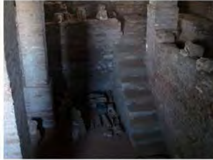
DSC06259.JPG, Inappropriate/Inexistent Site Drainage, Royal City
