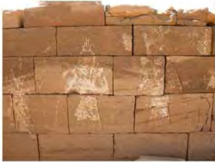
DSCN4084.JPG, Naqaa, Amun Temple, Exposure and Deterioration of Ancient Plasters, Degradation of Stone/Masonry Elements
