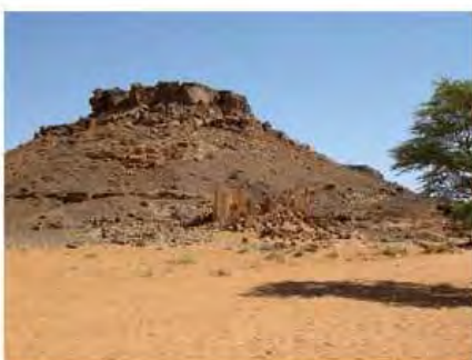
DSCN4137.JPG, Naqaa, Temple F, Site Wide View, Structural Instability of Walls/Collapse of Archaeological Features
