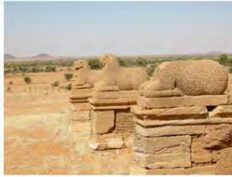
DSCN4133.JPG, Naqaa, Amun Temple, Exposure and Deterioration of Ancient Plasters
