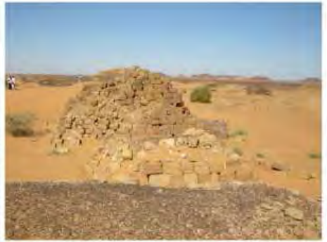
DSCN3850.JPG, Structural Deterioration of Pyramids, Southern Cemetery
