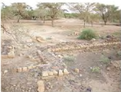
DSCN3950.JPG, Structural Instability of Walls/Collapse of Archaeological Features, Degradation of Stone/Masonry Elements, Vegetation Damage, Royal City
