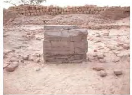
DSCN3970.JPG, Structural Instability of Walls/Collapse of Archaeological Features, Degradation of Stone/Masonry Elements, Royal City
