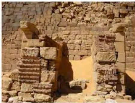
DSCN3763.JPG, Incoherent Repair Methods and Poor Craftsmanship, Northern Cemetery
