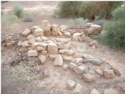
DSCN3944.JPG, Structural Instability of Walls/Collapse of Archaeological Features, Vegetation Damage, Royal City
