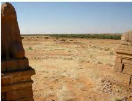
DSCN4076.JPG, Naqaa, Amun Temple, Exposure and Deterioration of Ancient Plasters
