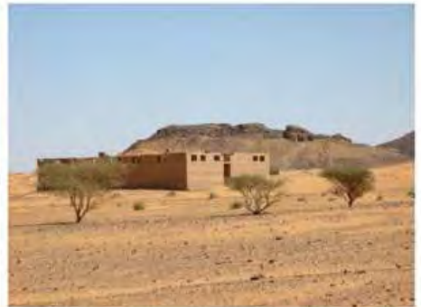
DSCN3812.JPG, Redundant/Inappropriate Visitor Infrastructure, Southern Cemetery
