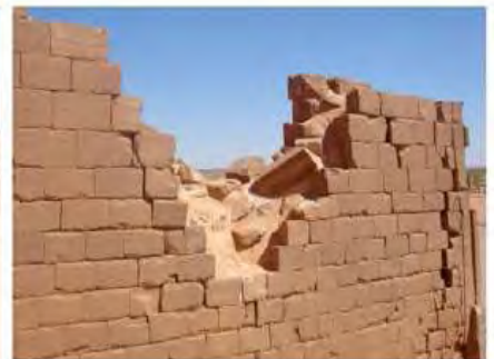
DSC06209.JPG, Musawwarat - Great Enclosure, Restoration Works
