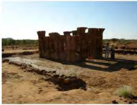
DSCN4018.JPG, The Kiosk - Naqaa, Naqaa, Degradation of Stone/ Masonry Elements, Inappropriate/Inexistent Site Drainage
