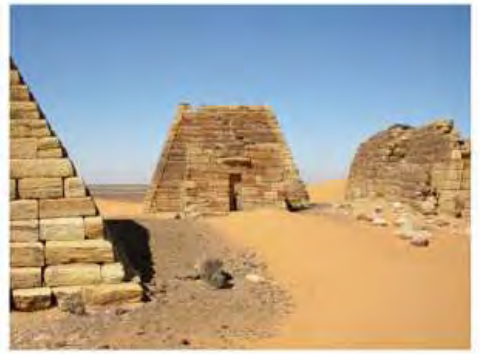
DSCN3746.JPG, Public Safety Hazard, Northern Cemetery
