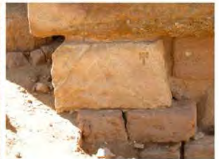
DSCN4121.JPG, Naqaa, Amun Temple, Exposure and Deterioration of Ancient Plasters, Degradation of Stone/Masonry Elements
