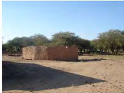
DSC06263.JPG, Redundant/Inappropriate Visitor Infrastructure, Royal City
