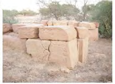
DSCN3931.JPG, Structural Instability of Walls/Collapse of Archaeological Features, Degradation of Stone/Masonry Elements, Inappropriate/Inexistent Site Drainage, Vegetation Damage, Royal City
