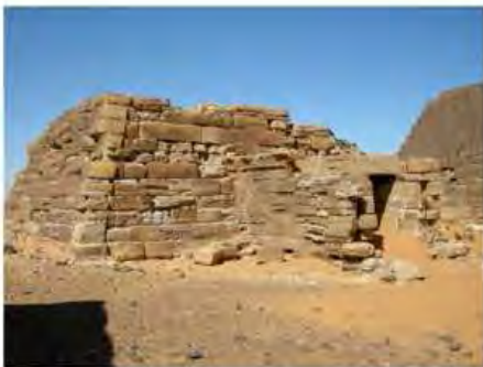
DSCN3726.JPG, Degradation of Stone/Masonry Elements, Northern Cemetery
