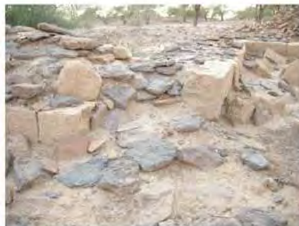
DSCN3948.JPG, Structural Instability of Walls/Collapse of Archaeological Features, Degradation of Stone/Masonry Elements, Royal City
