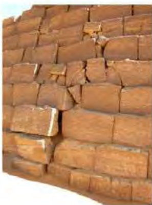
DSCN3741.JPG, Structural Deterioration of Pyramids, Northern Cemetery
