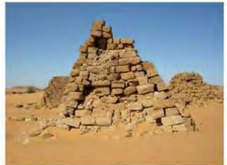
DSCN3859.JPG, Structural Deterioration of Pyramids, Southern Cemetery
