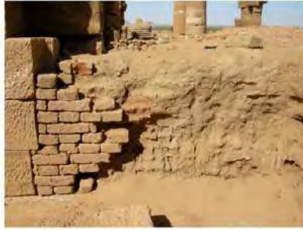
DSCN4110.JPG, Naqaa, Amun Temple, Deterioration of Ancient Mud Structures
