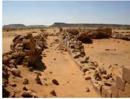
DSCN4177.JPG, Musawwarat - Great Enclosure, Structural Instability of Walls/Collapse of Archaeological Features, Structural Instability of Walls/Collapse of Archaeological Features
