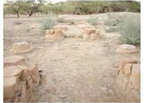
DSCN3934.JPG, Degradation of Stone/Masonry Elements, Structural Instability of Walls/Collapse of Archaeological Features, Inappropriate/Inexistent Site Drainage, Vegetation Damage, Royal City
