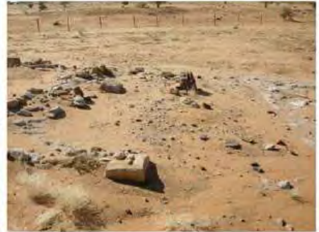
DSCN4065.JPG, Naqaa, Temple B200, Degradation of Stone/ Masonry Elements
