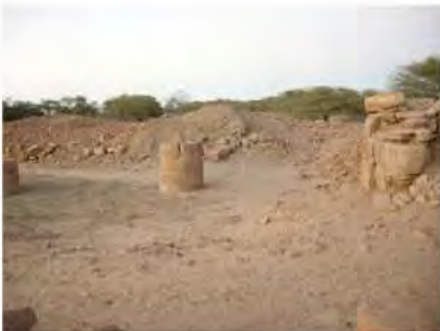
DSCN3959.JPG, Inappropriate Dumping of Excavation Spoils, Inappropriate/Inexistent Site Drainage, Royal City
