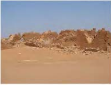
DSC06166.JPG, Musawwarat - Great Enclosure, Structural Instability of Walls/Collapse of Archaeological Features
