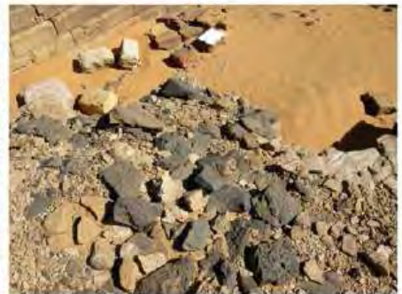
DSCN3731.JPG, Structural Deterioration of Pyramids, Northern Cemetery
