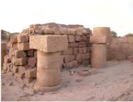
DSCN3980.JPG, Structural Instability of Walls/Collapse of Archaeological Features, Inappropriate Dumping of Excavation Spoils, Inappropriate/Inexistent Site Drainage, Royal City
