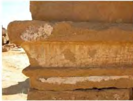
DSCN4073.JPG, Naqaa, Amun Temple, Exposure and Deterioration of Ancient Plasters
