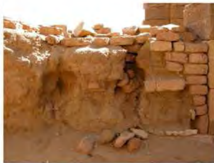
DSCN4103.JPG, Naqaa, Amun Temple, Deterioration of Ancient Mud Structures
