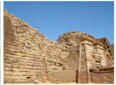
DSCN3770.JPG, Structural Deterioration of Pyramids, Northern Cemetery
