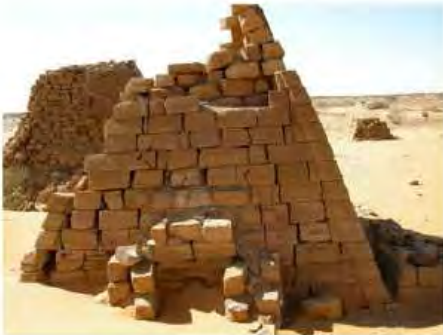
DSCN3857.JPG, Structural Deterioration of Pyramids, Southern Cemetery
