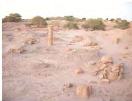
DSCN3984.JPG, Structural Instability of Walls/Collapse of Archaeological Features, Inappropriate Dumping of Excavation Spoils, Inappropriate/Inexistent Site Drainage, Royal City
