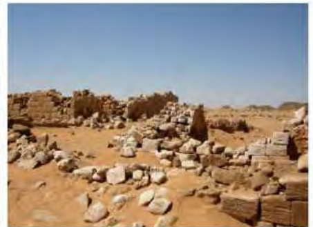
DSCN4169.JPG, Musawwarat - Great Enclosure, Structural Instability of Walls/Collapse of Archaeological Features, Degradation of Stone/Masonry Elements, Structural Instability of Walls/Collapse of Archaeological Features, Salt Crystallization
