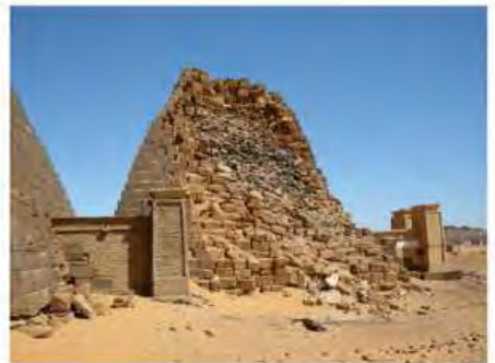
DSCN3803.JPG, Structural Deterioration of Pyramids, Southern Cemetery
