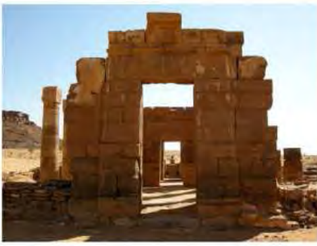
DSCN4088.JPG, Naqaa, Amun Temple, Exposure and Deterioration of Ancient Plasters
