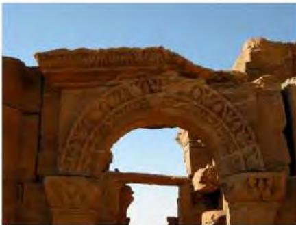
DSCN4017.JPG, The Kiosk - Naqaa, Naqaa, Structural Instability of Walls/Collapse of Archaeological Features
