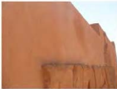
DSC06180.JPG, Musawwarat - Great Enclosure, Restoration Works
