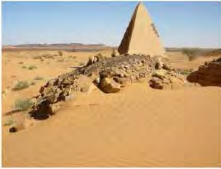
DSCN3845.JPG, Structural Deterioration of Pyramids, Southern Cemetery
