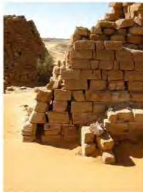
DSCN3858.JPG, Structural Deterioration of Pyramids, Southern Cemetery
