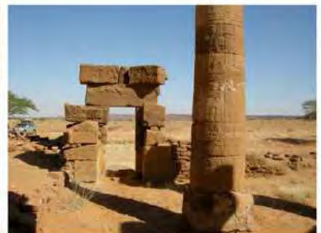
DSCN4099.JPG, Naqaa, Amun Temple, Degradation of Stone/Masonry Elements, Exposure and Deterioration of Ancient Plasters
