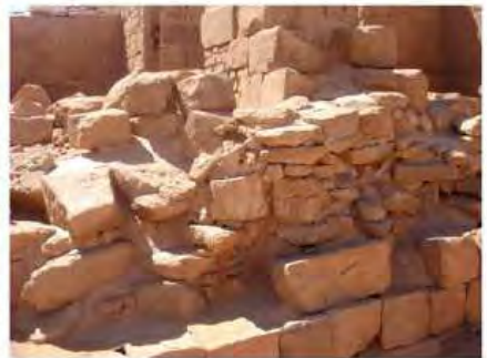
DSC06200.JPG, Musawwarat - Great Enclosure, Restoration Works
