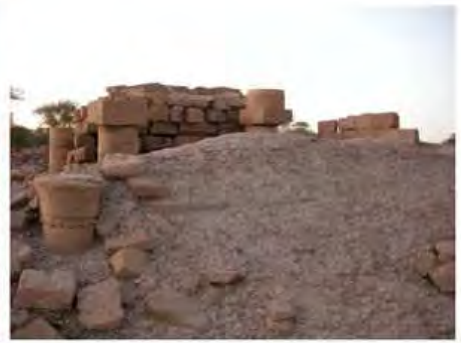
DSCN3979.JPG, Inappropriate Dumping of Excavation Spoils, Structural Instability of Walls/Collapse of Archaeological Features, Royal City
