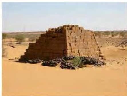
DSCN3865.JPG, Structural Deterioration of Pyramids, Southern Cemetery
