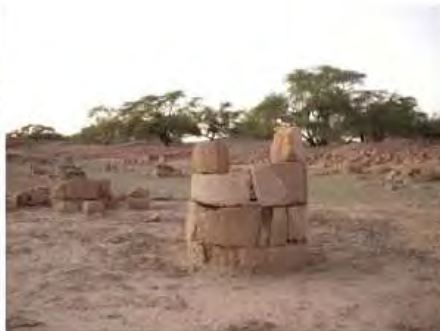
DSCN3960.JPG, Degradation of Stone/Masonry Elements, Structural Instability of Walls/Collapse of Archaeological Features, Inappropriate/Inexistent Site Drainage, Royal City
