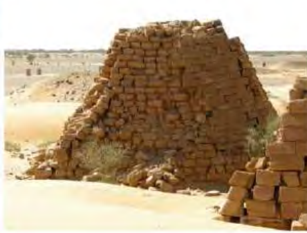
DSCN3855.JPG, Structural Deterioration of Pyramids, Southern Cemetery
