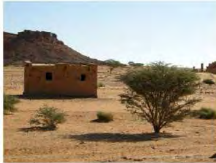
DSCN4057.JPG, Naqaa, Site Wide View, Redundant/Inappropriate Visitor Infrastructure
