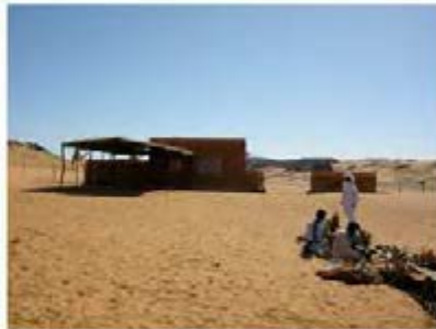
DSCN3703.JPG, Redundant/Inappropriate Visitor Infrastructure, Northern Cemetery
