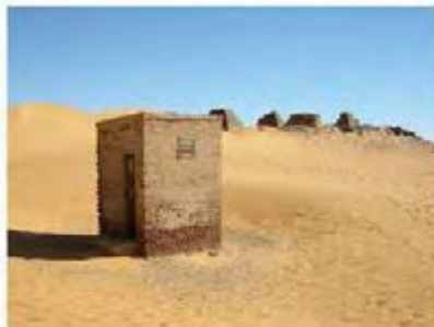
DSCN3706.JPG, Redundant/Inappropriate Visitor Infrastructure, Northern Cemetery
