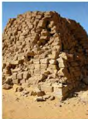
DSCN3862.JPG, Structural Deterioration of Pyramids, Southern Cemetery
