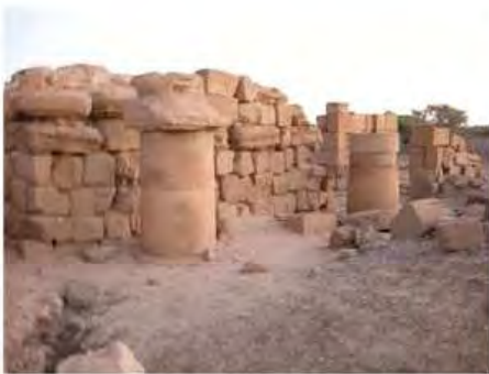
DSCN3986.JPG, Inappropriate Dumping of Excavation Spoils, Inappropriate/Inexistent Site Drainage, Royal City
