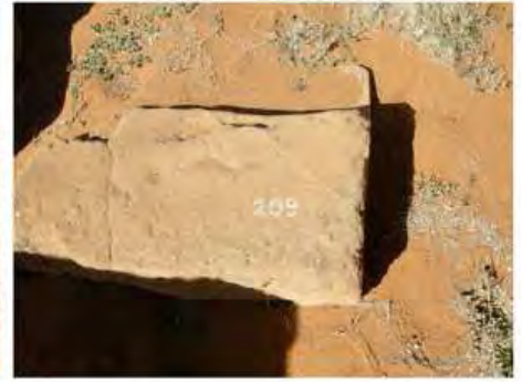
DSCN4116.JPG, Naqaa, Amun Temple, Inappropriate/Inexistent Site Drainage
