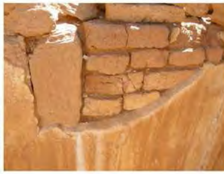
DSCN4113.JPG, Naqaa, Amun Temple, Exposure and Deterioration of Ancient Plasters
