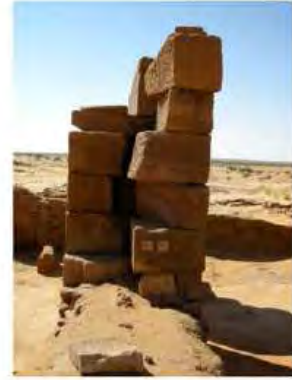
DSCN4118.JPG, Naqaa, Amun Temple, Structural Instability of Walls/Collapse of Archaeological Features
