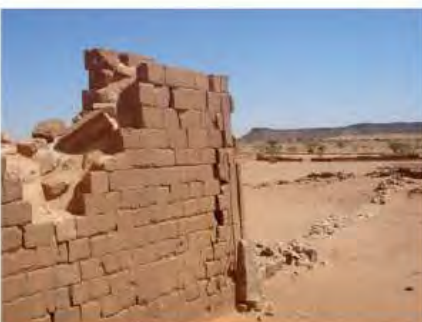
DSC06210.JPG, Musawwarat - Great Enclosure, Restoration Works
