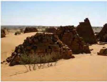
DSCN3842.JPG, Structural Deterioration of Pyramids, Southern Cemetery
