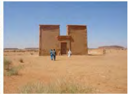
DSC06215.JPG, Musawwarat - Re-erected Lion Temple, Restoration Works
