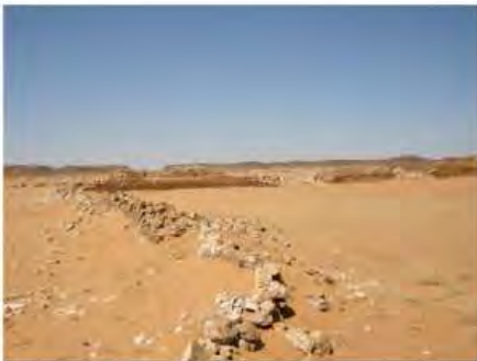
DSCN4167.JPG, Musawwarat - Great Enclosure, Structural Instability of Walls/Collapse of Archaeological Features
