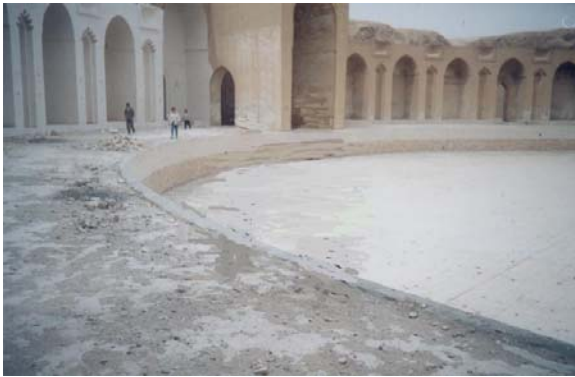
(Figure # 24) The circular basin inside The Caliphal palace.
