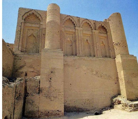
(Figure # 31) One of Al-Ma'shuq Palace facades.
