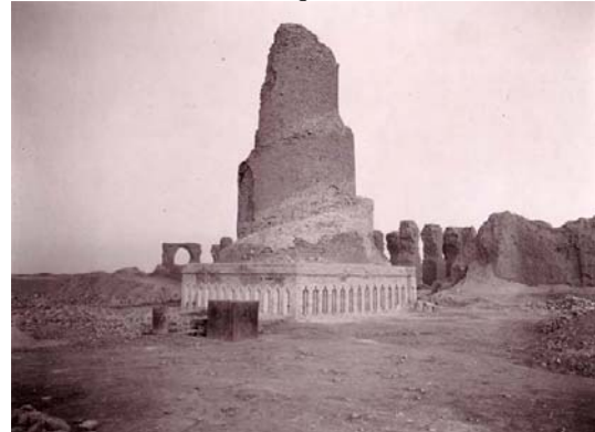
(Figure # 21) Spiral minaret of Abu Dulaf Mosque (before conservation)
