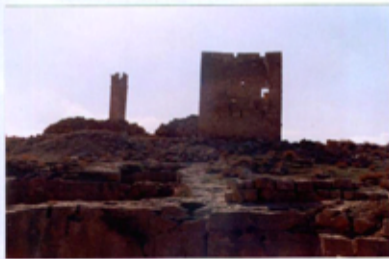
Detail of the reservoirs, one still roofed with arches and slabs
