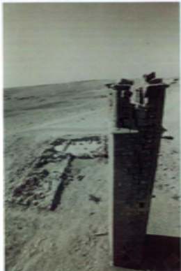
Aerial View of The Tower with its Church to the South
