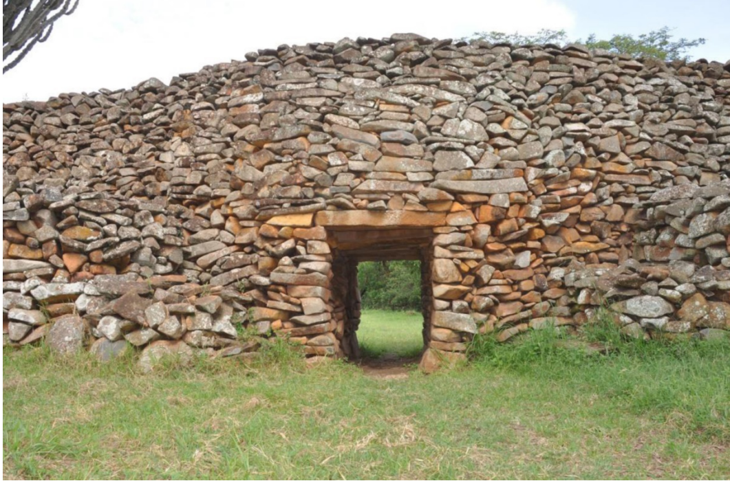
Main entrance to K'Ochieng' enclosure
