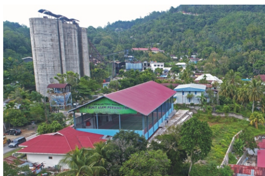
Image.4.1 (L) Construction of new structures in the Coal Processing Plant Compound
