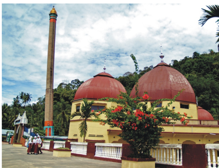
Image.4.4 Major structural changes in Kubang Sirakuak Power Plant (now a Nurul Iman Mosque). Authentic vestiges of this property include the chimney and underground boiler chamber (A4.2)
