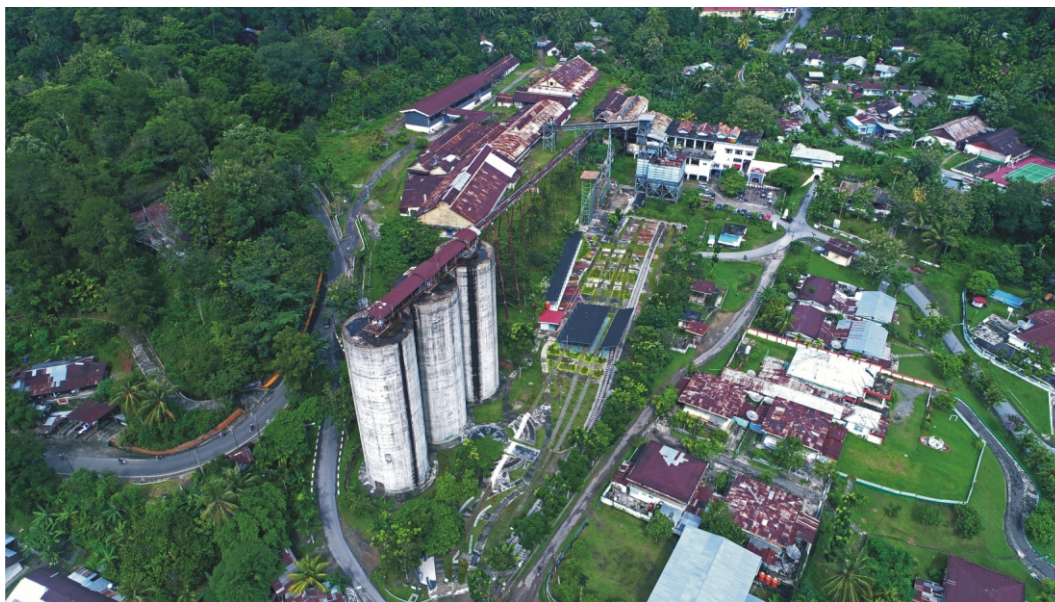
Image.4.7 Some parts of the railway emplacement in the Coal Processing Plant Compound were covered and converted into a public space ( Taman Silo )
