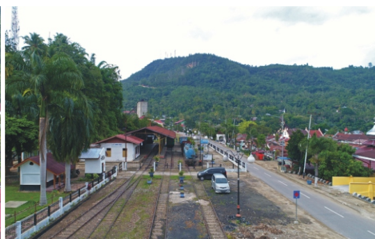
Image.4.2 (R) Construction of new road near Sawahlunto Train Station
