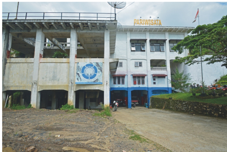
Image.4.6 Adaptive re-use of part of a building in the Coal Processing Plant Compound which now functions as local Tourism Office
