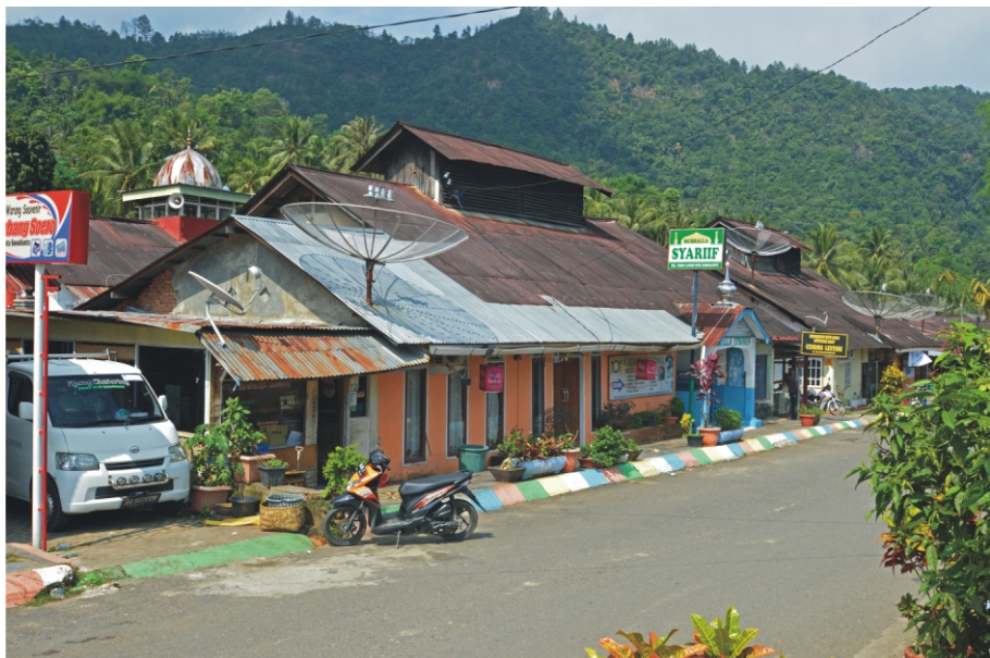
Image.4.22 Additional rooms were constructed to accommodate new tenants at the Tangsi Baru area (A5.2.b)
