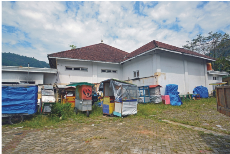
Image.4.23 Many street vendors store their cart recklessly behind the Assembly Hall (A5.5.b)
