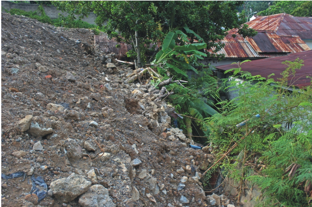
Image.4.13 Landslide behind W-29 (A5.1.d) in 2016, one of the significant objects within the Mining Administrative Compound
