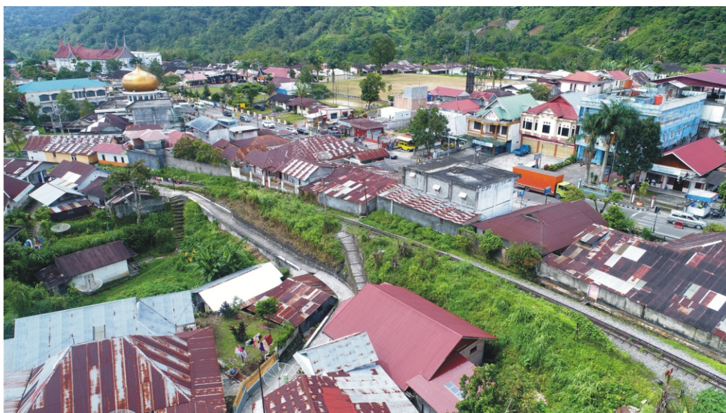
Image.4.3 Construction of houses very near to the railway at Padang Pandjang Train Station
