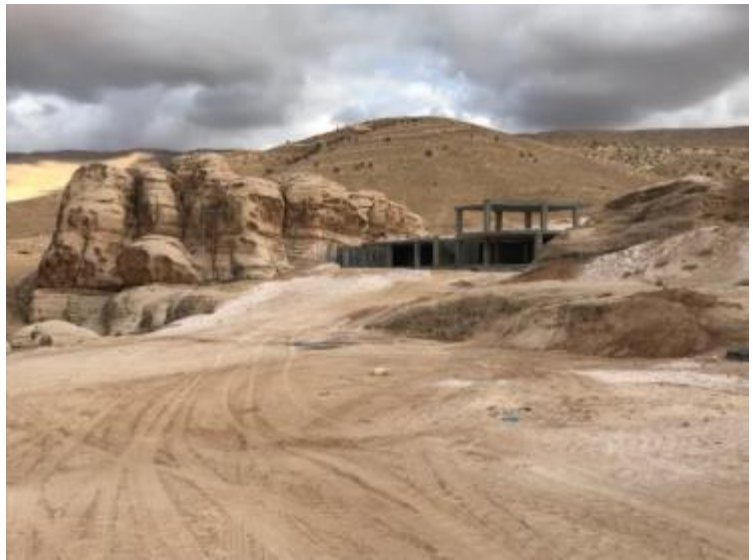
Fig 14 Ongoing Construction at the Eco Village
