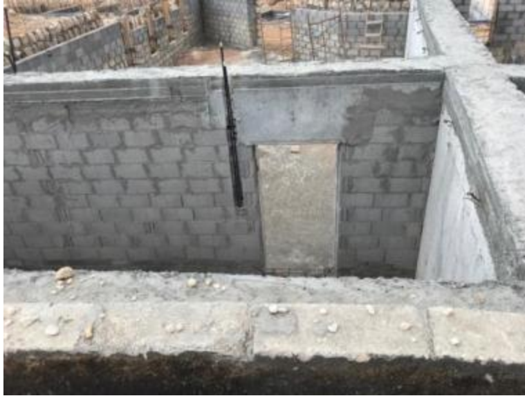
Fig 12 Ongoing Construction at the Heritage Village
