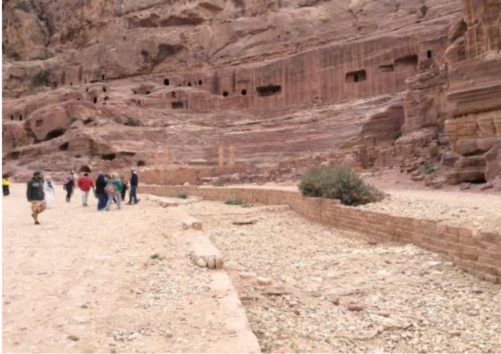
Fig 19 Petra Theatre with Main Trail and Wadi Musa showing retaining walls and concrete capping. Photo: Tom Hassall.
