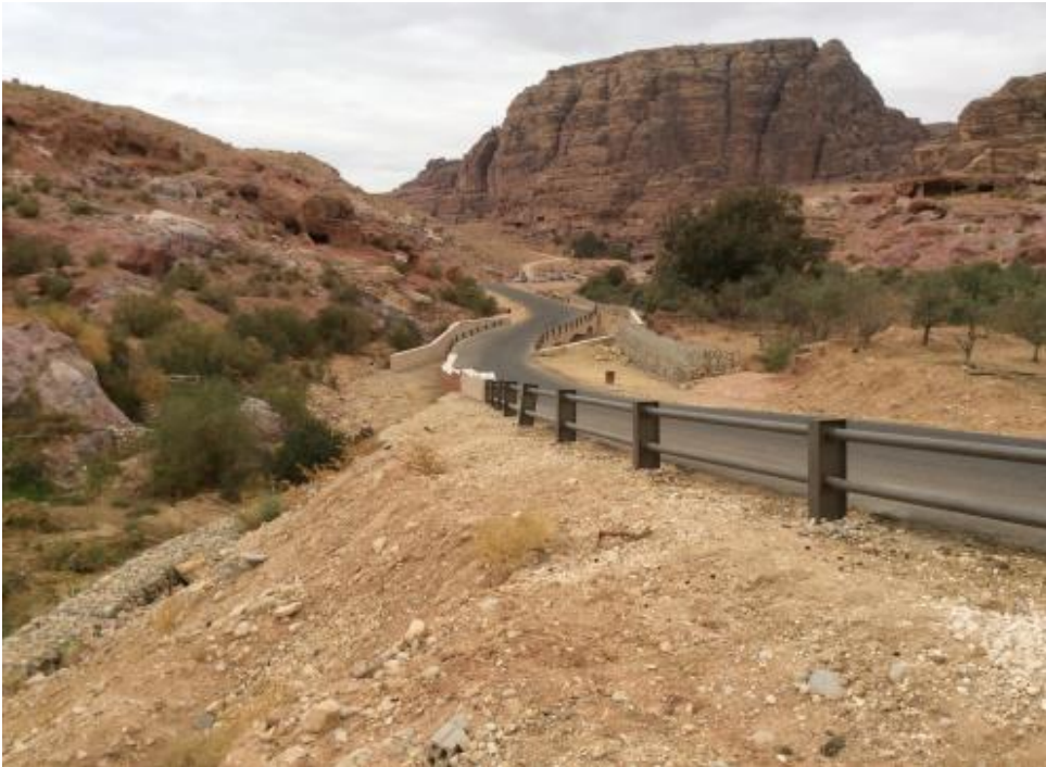
Fig 26: Petra Wadi Turkmenia with new Back Road Terminus with shelters and turning circle. Photo: Tom Hassall
