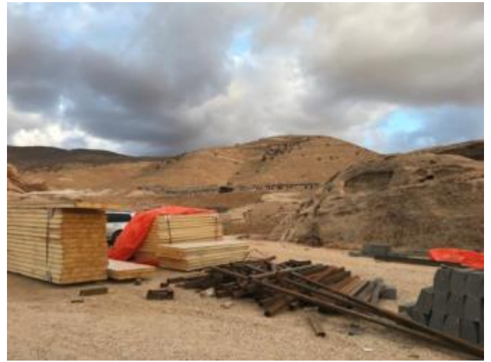
Fig 11 Ongoing Construction at the Heritage Village
