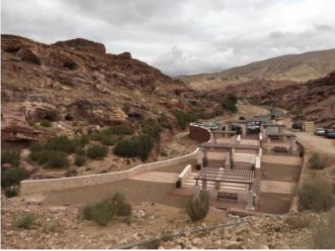
Fig 4 Back Road/Shelters and Parking
