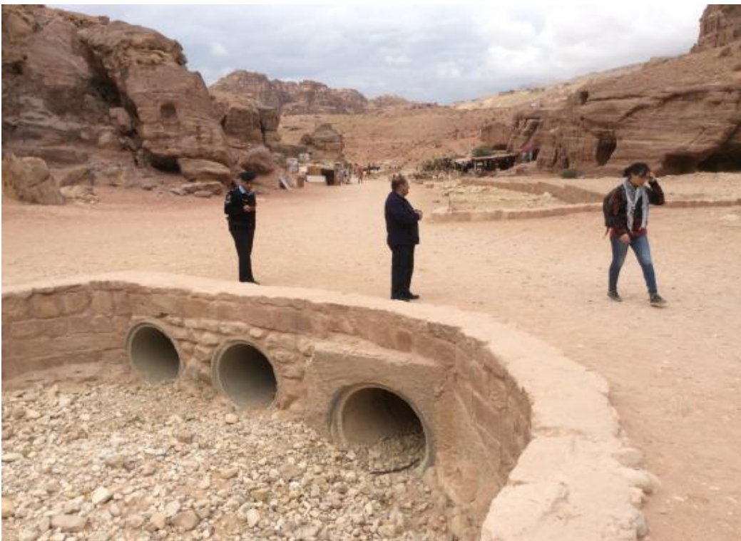
Fig 18 Petra Main Trail and Wadi Musa showing bridge and concrete drain pipes and retaining walls. Photo: Tom Hassall.
