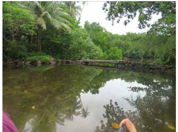
Fig 18: Another one of the later bridges
