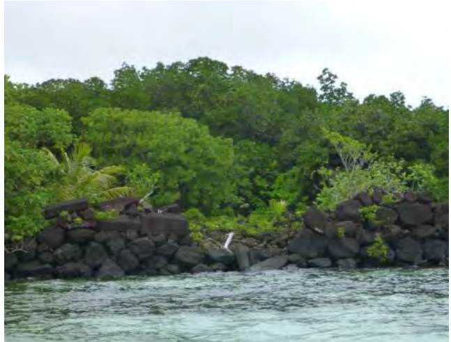
To reinstate sea defences and restrict internal bulk fill erosion
