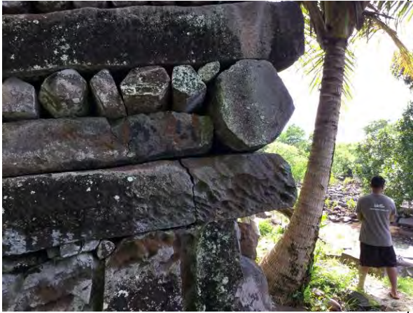
Fig 13: Cracked stone with section missing below – this will need propping
