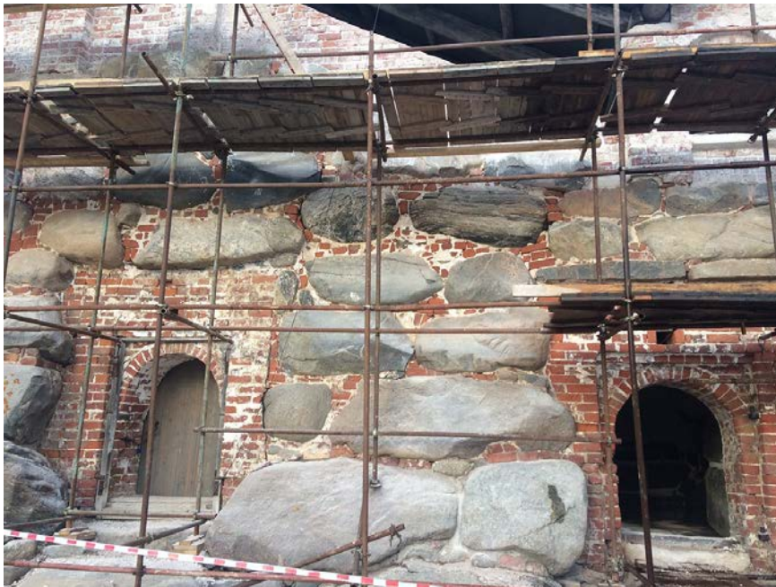
Fig. 4d: The basement of the gallery-passageway within Solovetsky Monastery Complex
