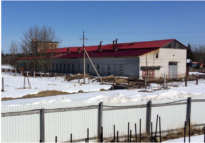
Fig. 8b: The diesel power station on Solovetsky Island
