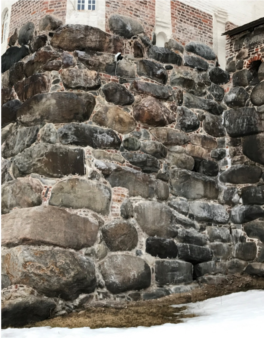
Fig. 6b: Tower after cleaning and repointing
