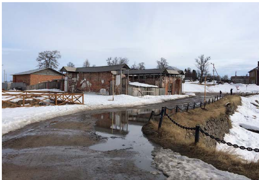
Fig. 8a: The hydro-electric power station on Solovetsky Island
