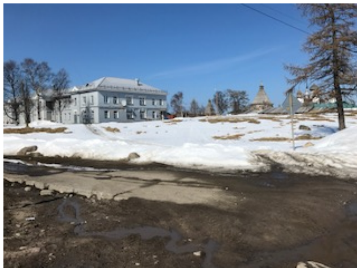
Fig. 11: Gulag-era hospital building
