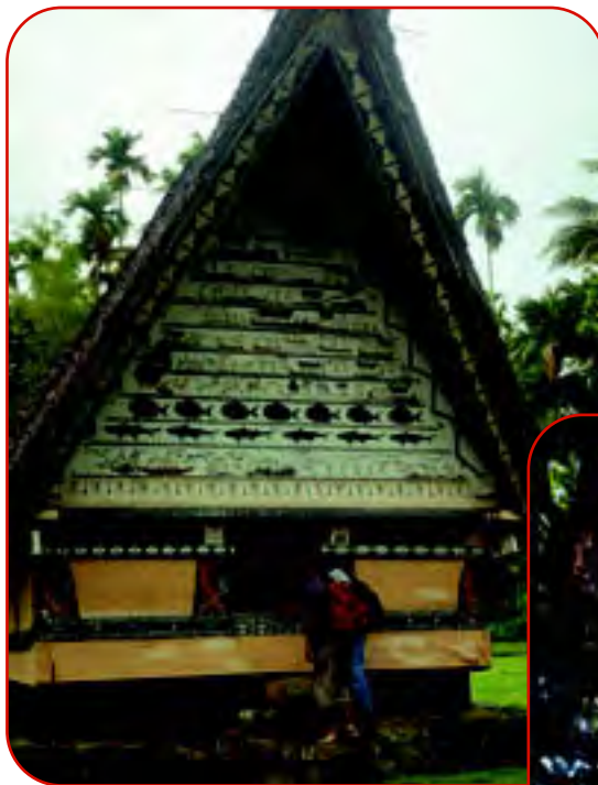
The Bai of Airai, which is the last traditional meeting house remaining on Babeldoab, Palau.
