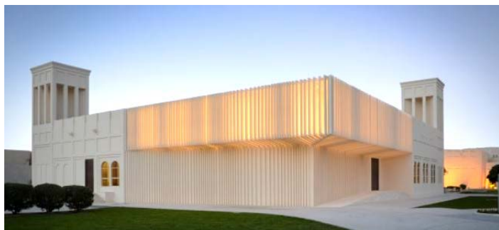
Headquarters of Arab Regional Centre for World Heritage
