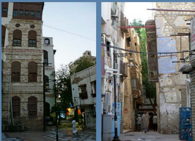
Ph.31: Bayt Naseef: structure with tiered teak beams – F. Cristofoli, 2009 Ph.32: The effect of poorly laid foundations and unstable soil – F. Cristofoli, 2009
