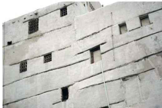
Ph.186: Embedded wooden beams – Ecole d'Avignon, 2006
