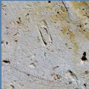
Ph.33: Coral stone in masonry with dark brown clay mortar – F. Cristofoli, 2009
