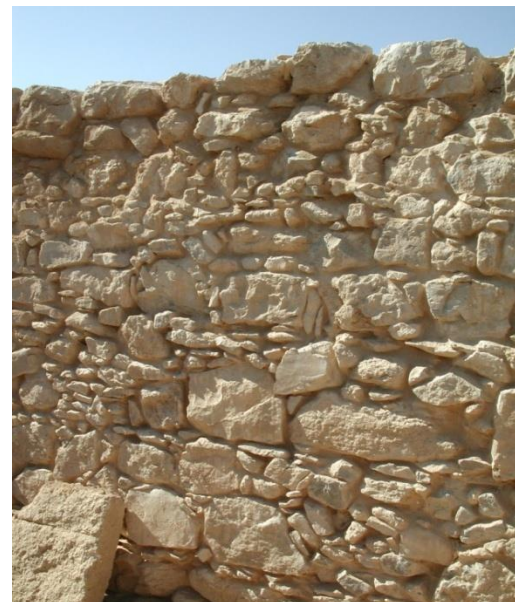
The Restoration work in Tabula Church 2005
