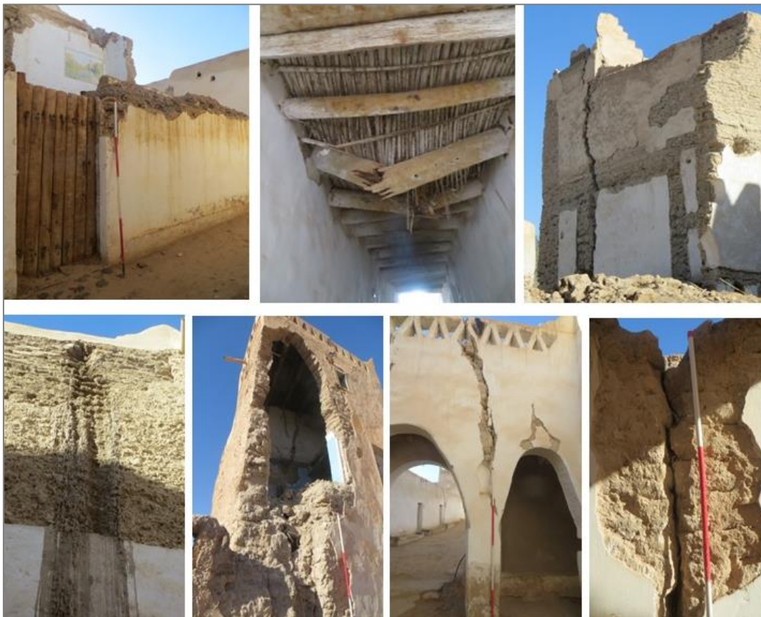
Examples of damage due to heavy rain in December 2017
