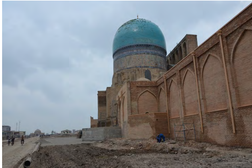
Underpinning structures after lowering of ground level in 2015
