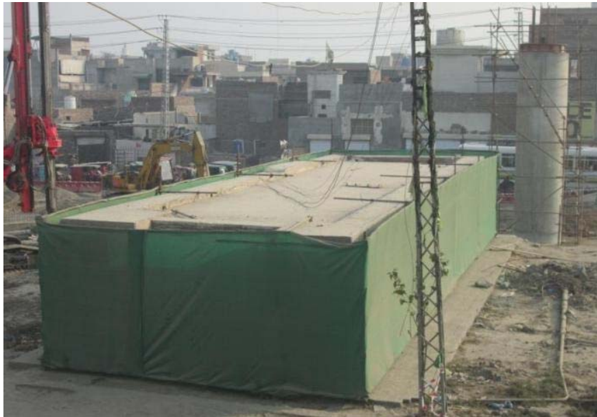
Bracing & Netting / Sheeting Arrangements at Hydraulic Tank
