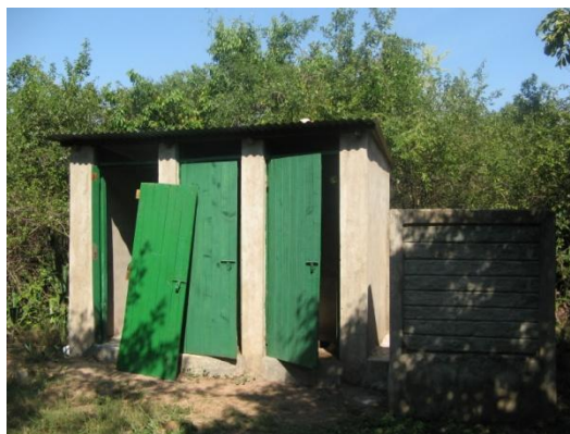
Plate 24 : Toilet door at ablution block in need of repair
