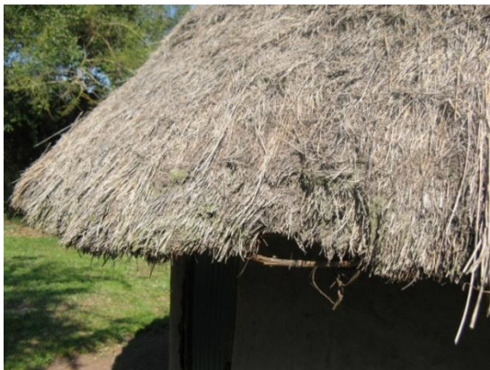
Plate 16: House in need of re-thatching smearing
