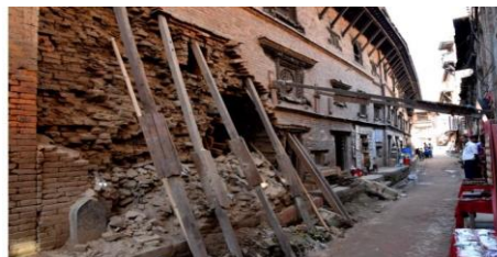
Emergency Shoring after earthquake at Pujarimath.
