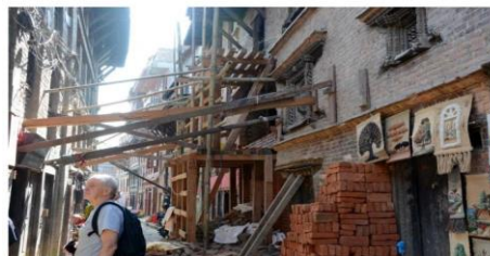
Shoring During Conservation at Pujarimath.
