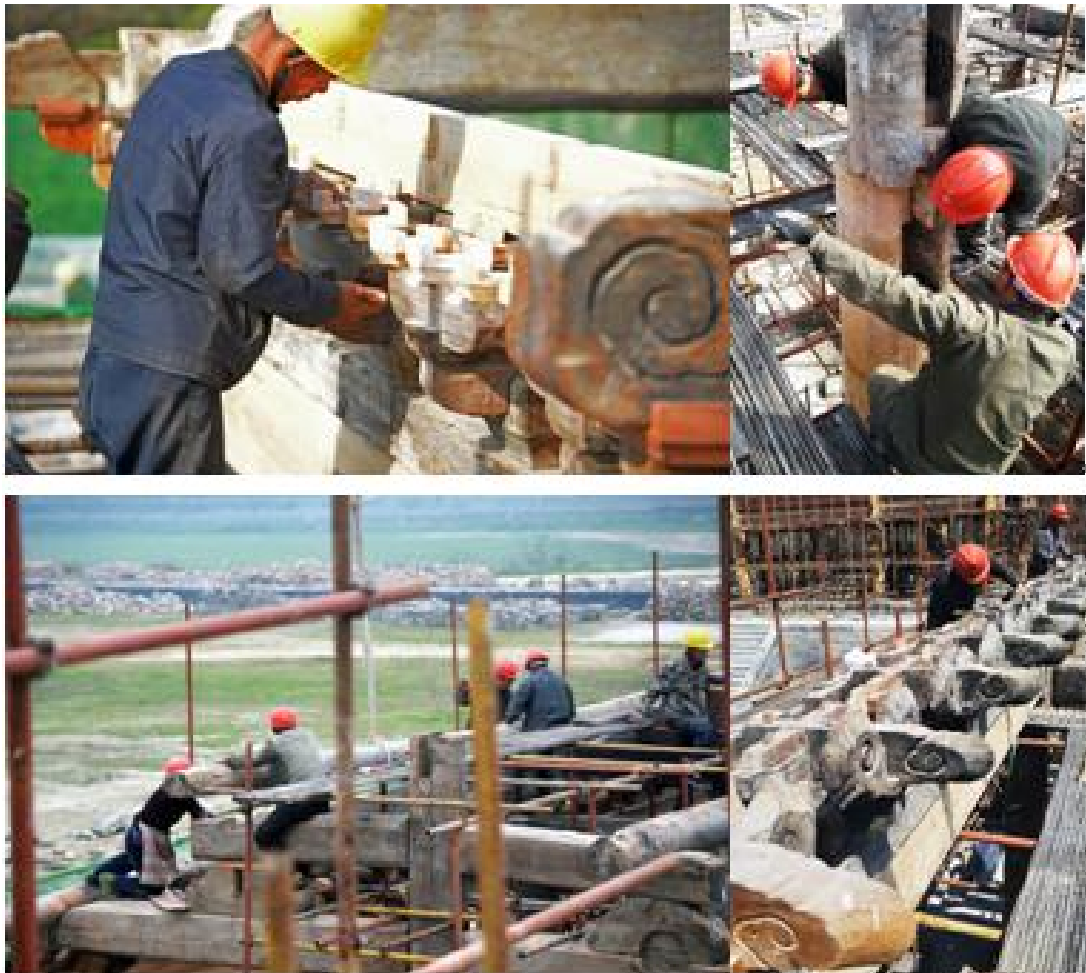
Photo 4. The re-installation of the middle court and buildings' main framework at the original site
