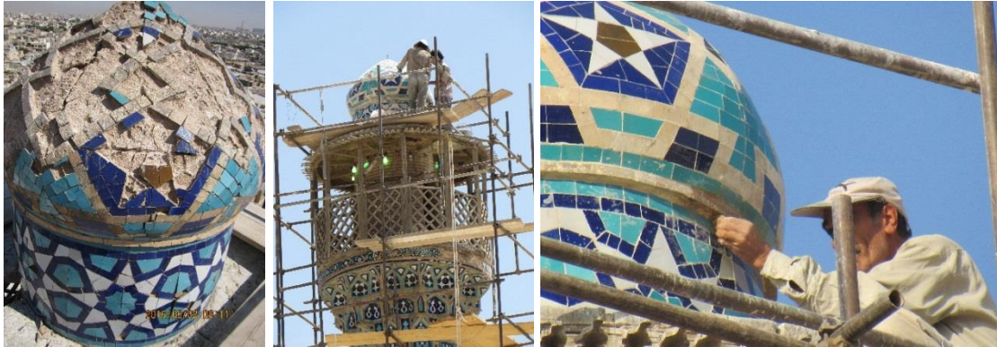
Figure 10. Restoration measure on the minarets' tiles
