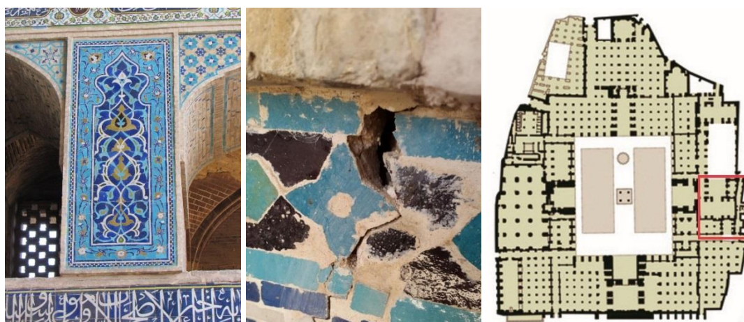
Figure 20. restoration and stabilization of decorative tiles on the facades of Mozafari Madrassah
