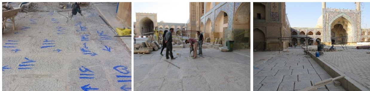
Figure 21. Slope correction of the inner-court and reorganization of pavements
