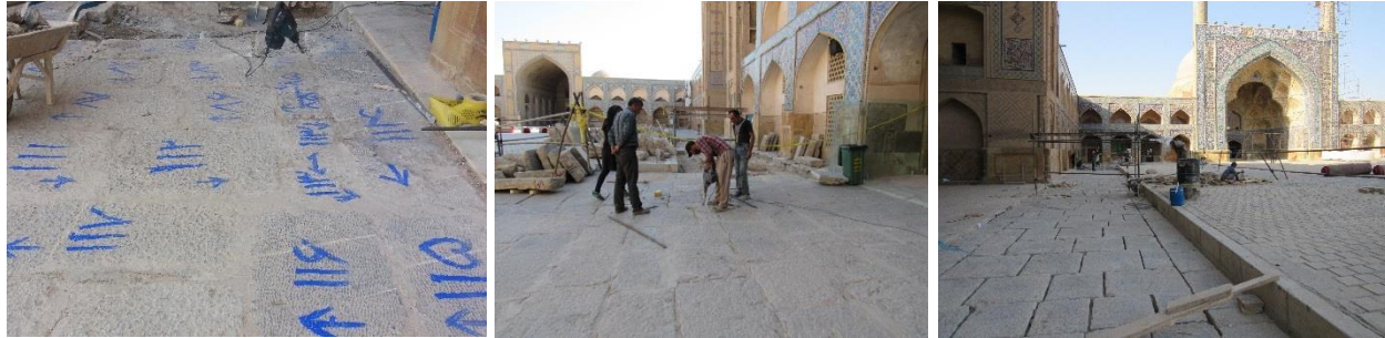
Figure 13. Slope correction of the inner-courtyard and reorganization of pavements
