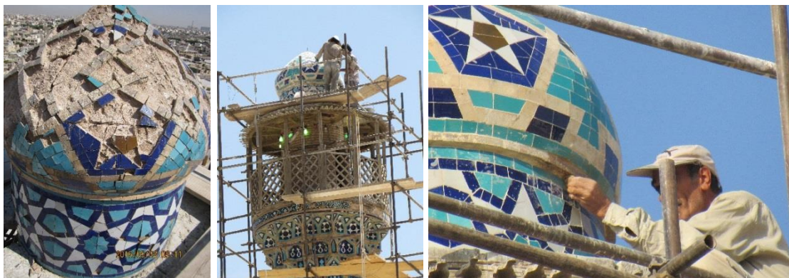
Figure 18. Restoration measure on the minarets' tiles
