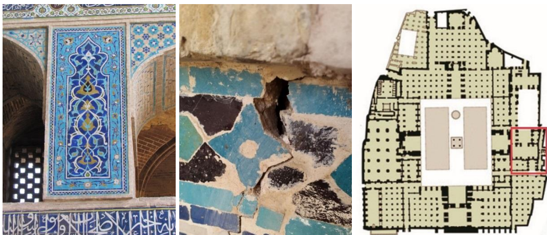
Figure 12. restoration and stabilization of decorative tiles on the facades of Mozafari Madrassah
