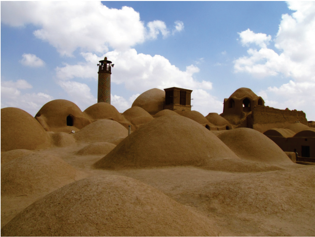
Kolombu and water cistern windcatcher
