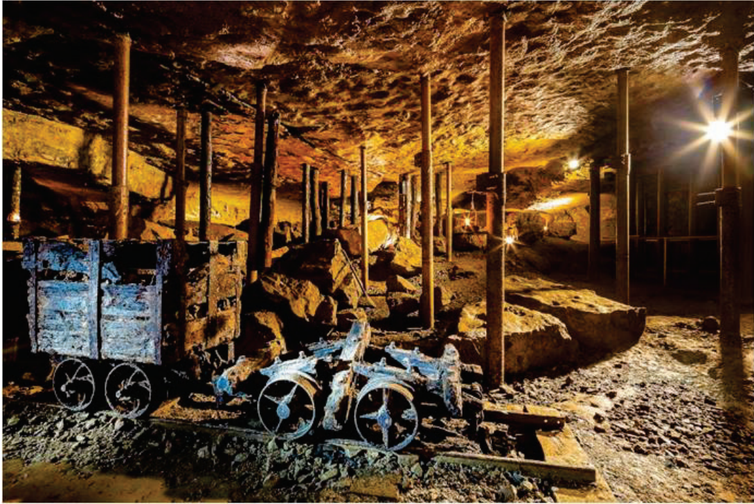
Single wooden pole supports
