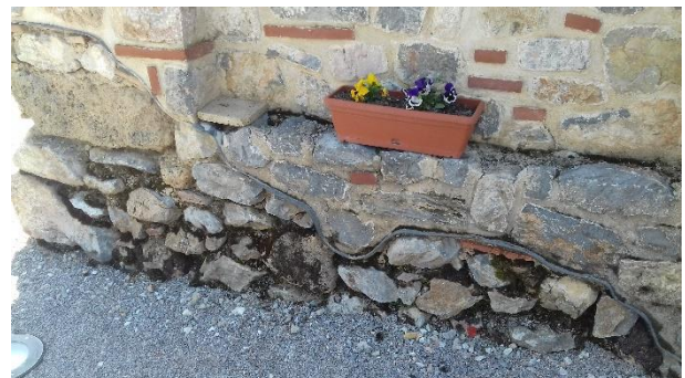
Separation of the wall of the reconstructed church from the original substructure, by a sheet of lead
