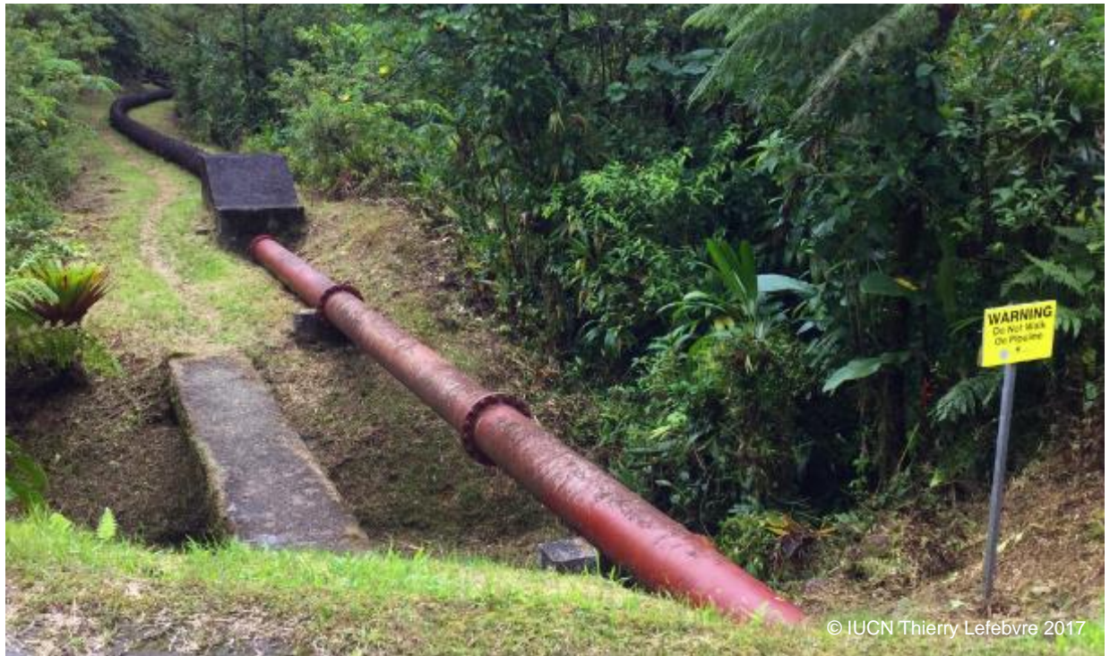
Photograph 5. Hydropower infrastructure near Freshwater lake
