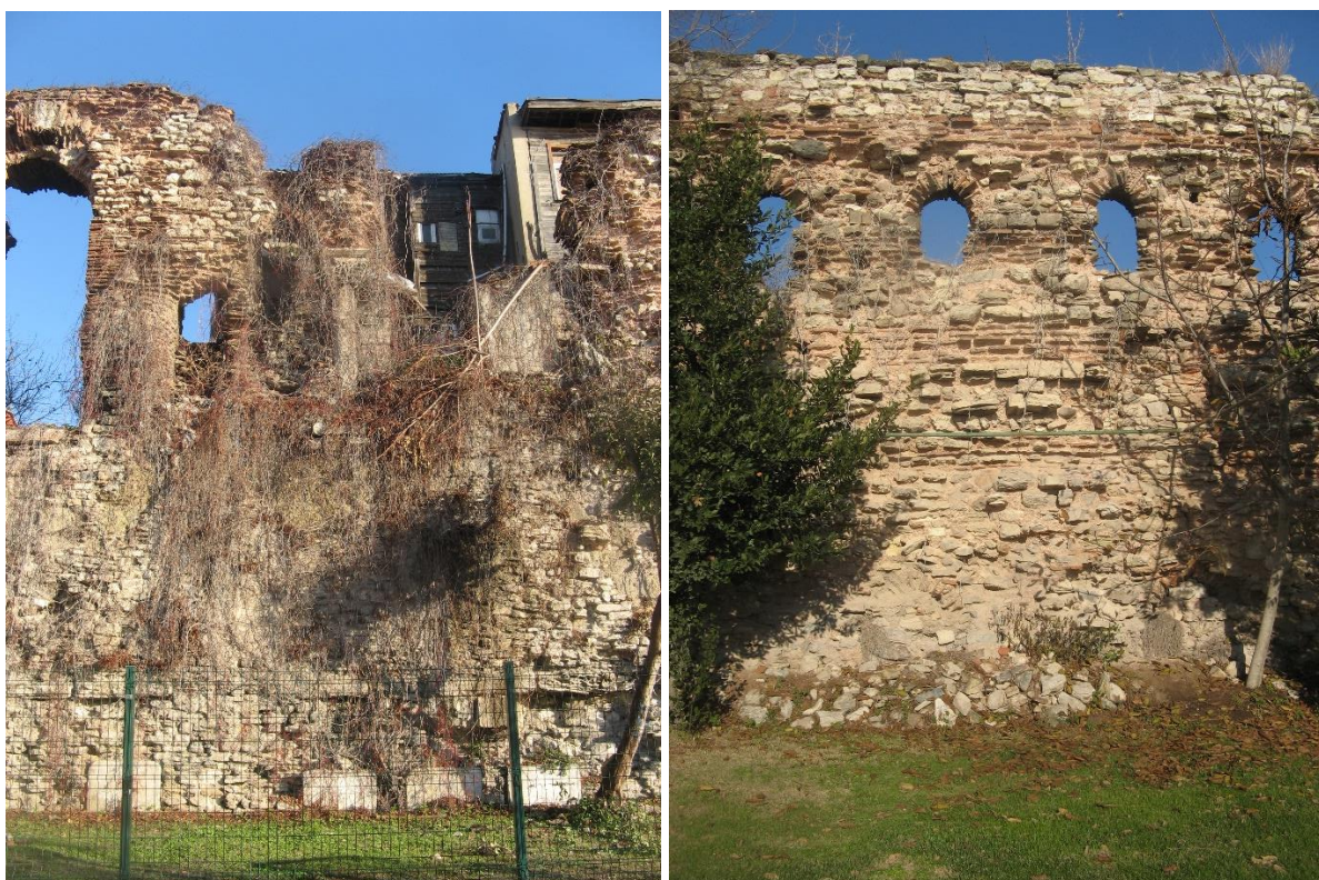
Fig 10 Bukoleon Palace, left, detail at left side of Fig 12; sea wall outside Kalyon Hotel showing deep erosion of mortar and debris at the foot of the wall
