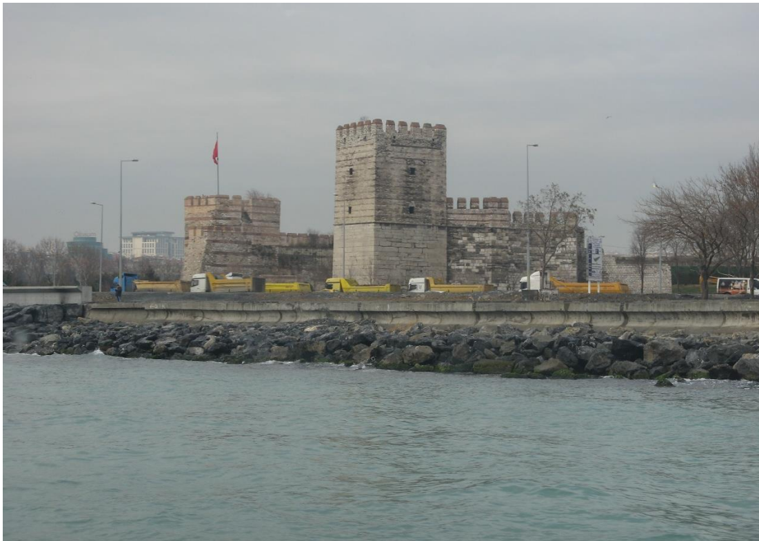
Fig 2 The Marble Tower from the sea, with the southern turret of the land wall beyond; the road is between the sea wall and the yellow trucks. To the left the extension of the sea wall is visible, slightly higher than the existing; further infill is anticipated in the foreground
