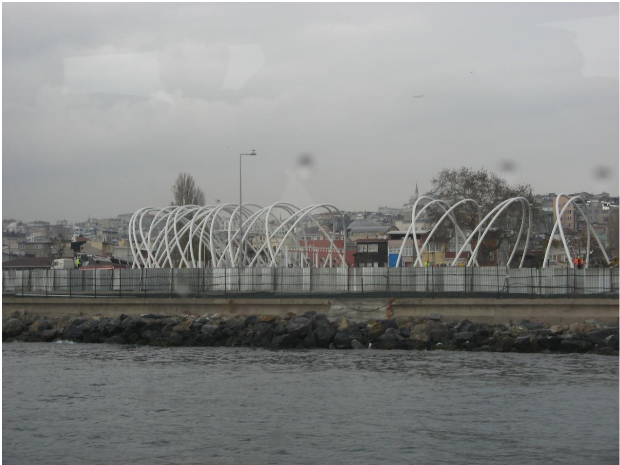
Fig 8 The toll plaza from the sea, slightly elevated to protect the tunnel mouth from tsunami waves; the hooped steel frames carry lighting and prevent over-height vehicles from entering the tunnel
