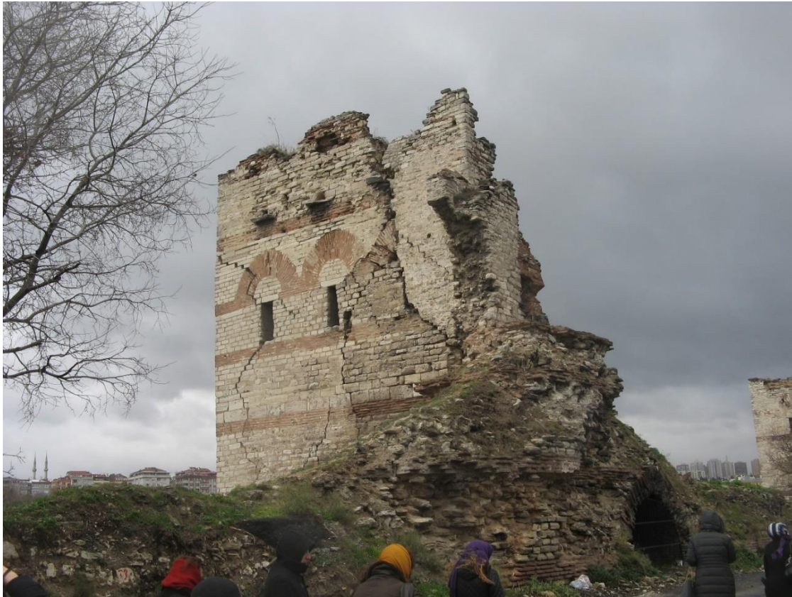
Fig 18 One of the bastions that has long been unstable (the large section to the right at high level is an ancient repair)
