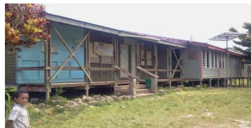
fig.7 Tingoa Health centre
