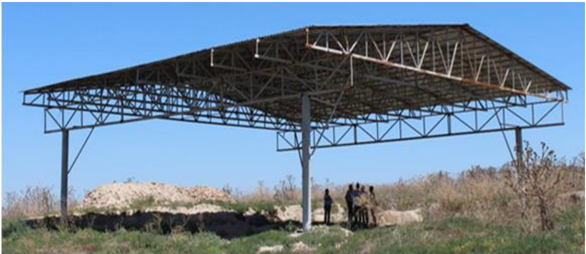
Shelter over excavation, 2016
