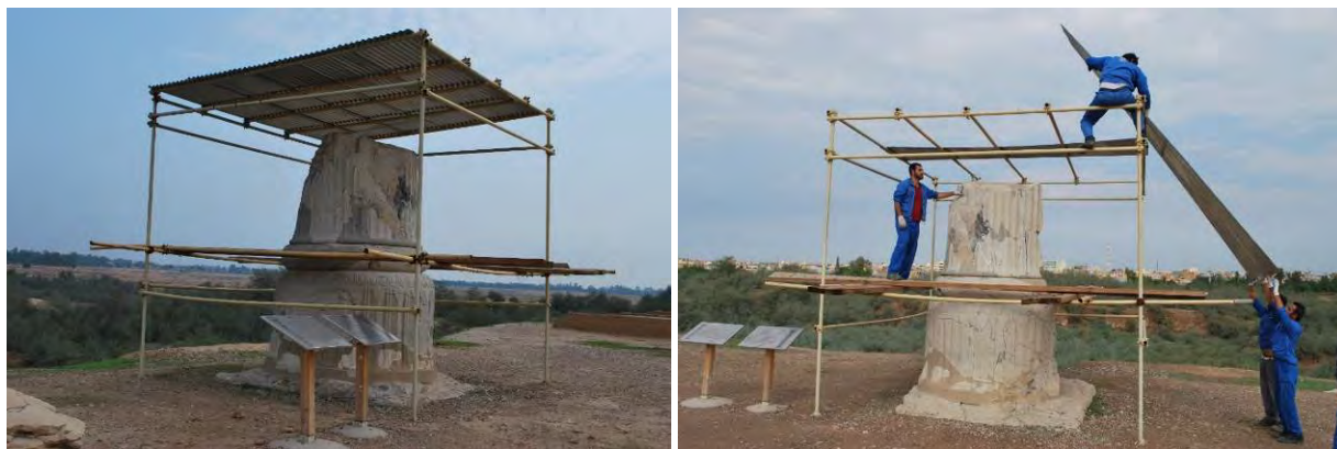
Figure 40. Temporary Covering of Achaemenid Columns in Apadana
