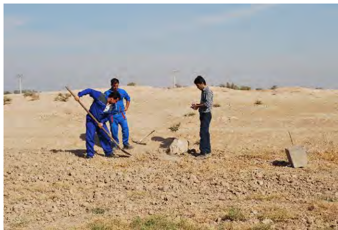
Figure 3. Placing cement piles in order to mark the boundaries of Ayadana
