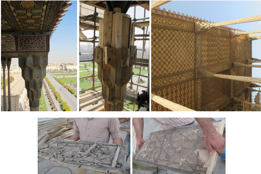
Figure 11. Restoration of decorative wooden elements
