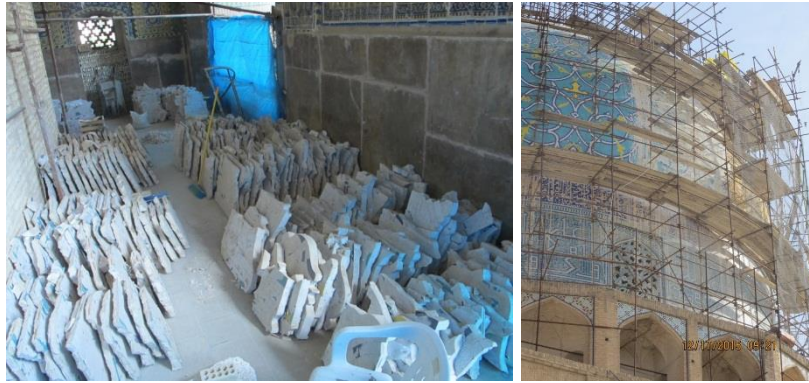
Figure 9. Reinforcement and restoration of the decoration tiles on Masjed-e Emam dome (left)- a part of installed tiles after restoration and reinforcement (right)
