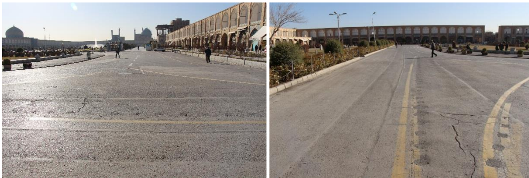
Figure 16. the Asphalt coverage of the square and its condition within the northern side- before reorganization of the site- ©Meydan Emam Base's Archive
