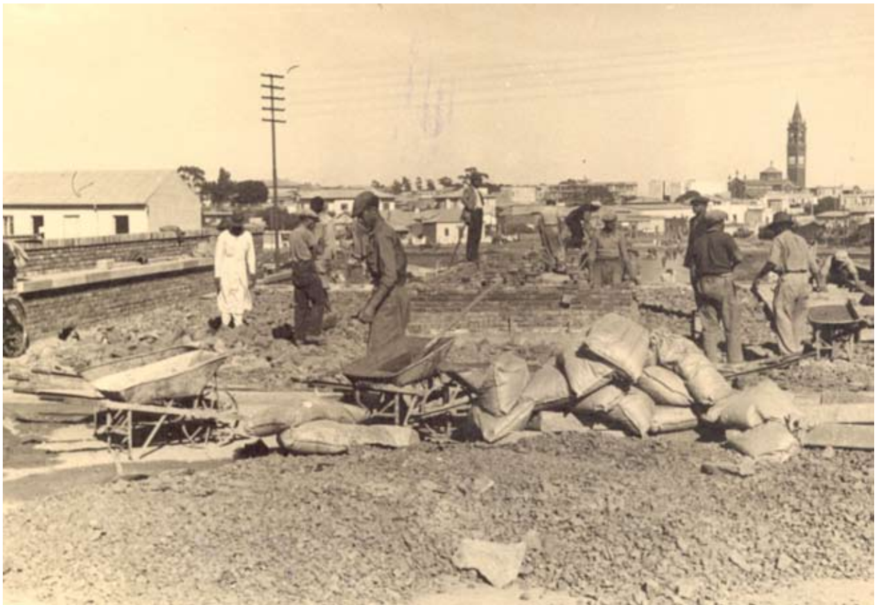
Fig 1.28: Eritrean bricklayers and construction workers building Mai Jab Jab foundation.
