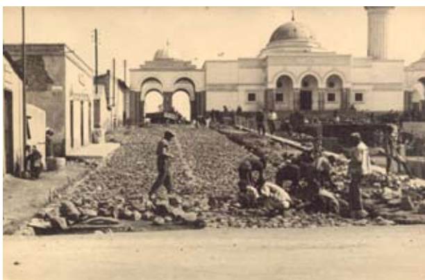
Fig 1.9-1.10: Eritrean and Italian labourers laying basalt blocks under the surface of new roads in Asmara's city centre.
