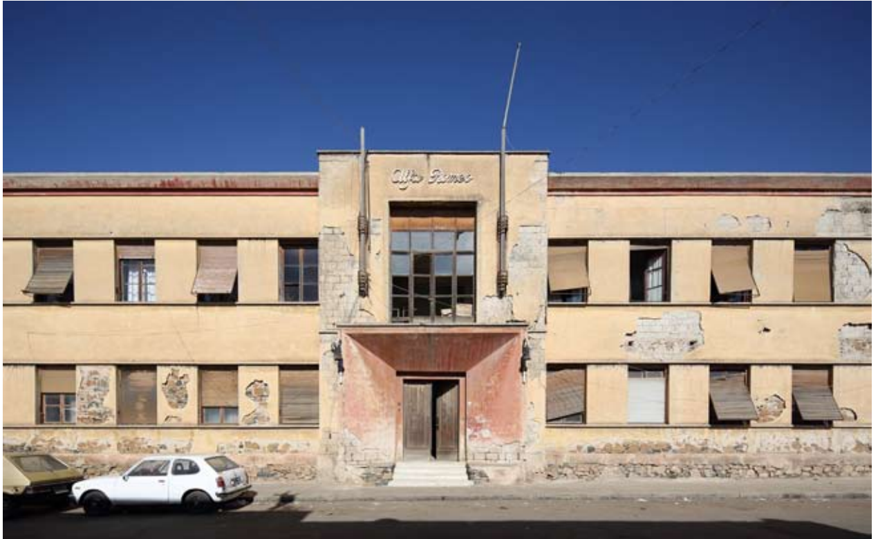
Figs 1.15 & 1.16: Former Società Anonima Alfa Romeo (SAAR) (1937) and a former villa both revealing behind their crumbling plaster the hollow concrete blocks used in their construction.
