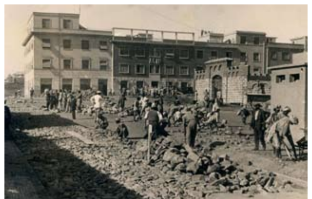
Fig 1.9-1.10: Eritrean and Italian labourers laying basalt blocks under the surface of new roads in Asmara's city centre.
