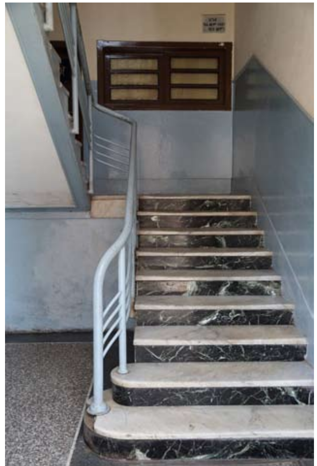
Figs 1.17 - 1.19: (left, bottom) marble polishing machine and (above and below) staircases in 1930s buildings in Asmara with treads and risers of different types of marble.
