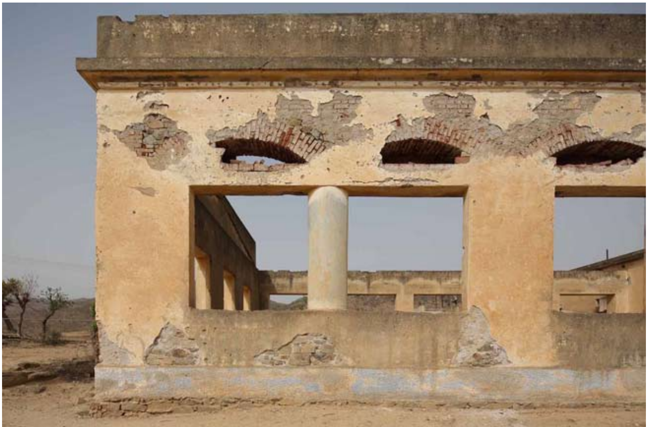
Fig 1.1-1.3: Ruin of a former water processing plant between Asmara and Massawa designed in a modernist style revealing the comparatively conventional building techniques and materials behind the plasterwork to create the desired modernist appearance defined by simple angular and geometric forms and an absence of ornamentation. This example outside the nominated property has been used to illustrate the point because the ruin reveals the underlying structure, which is rare in Asmara owing to the generally good state of conservation.
