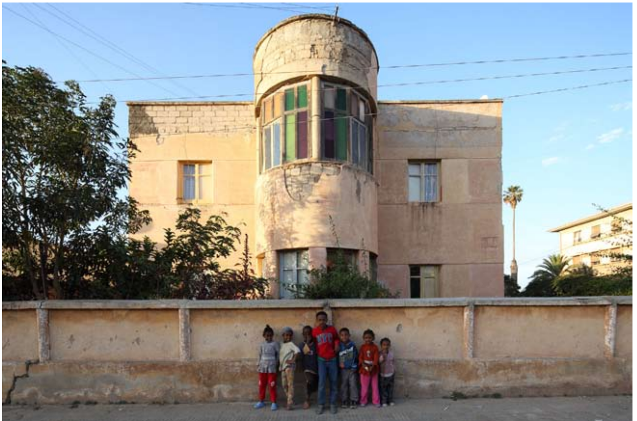
Figs 1.15 & 1.16: Former Società Anonima Alfa Romeo (SAAR) (1937) and a former villa both revealing behind their crumbling plaster the hollow concrete blocks used in their construction.
