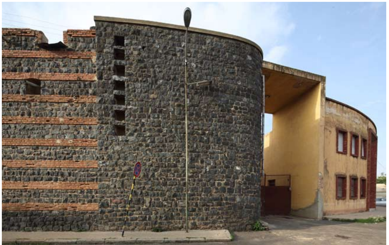
Fig 1.5 The Spinelli Store (late 1930s) showing the bands of basalt and brick combined with the angular and monumental reinforced concrete entrance arches. Similar building techniques can be found in Eritrea from the fourth century AD (see overleaf).
