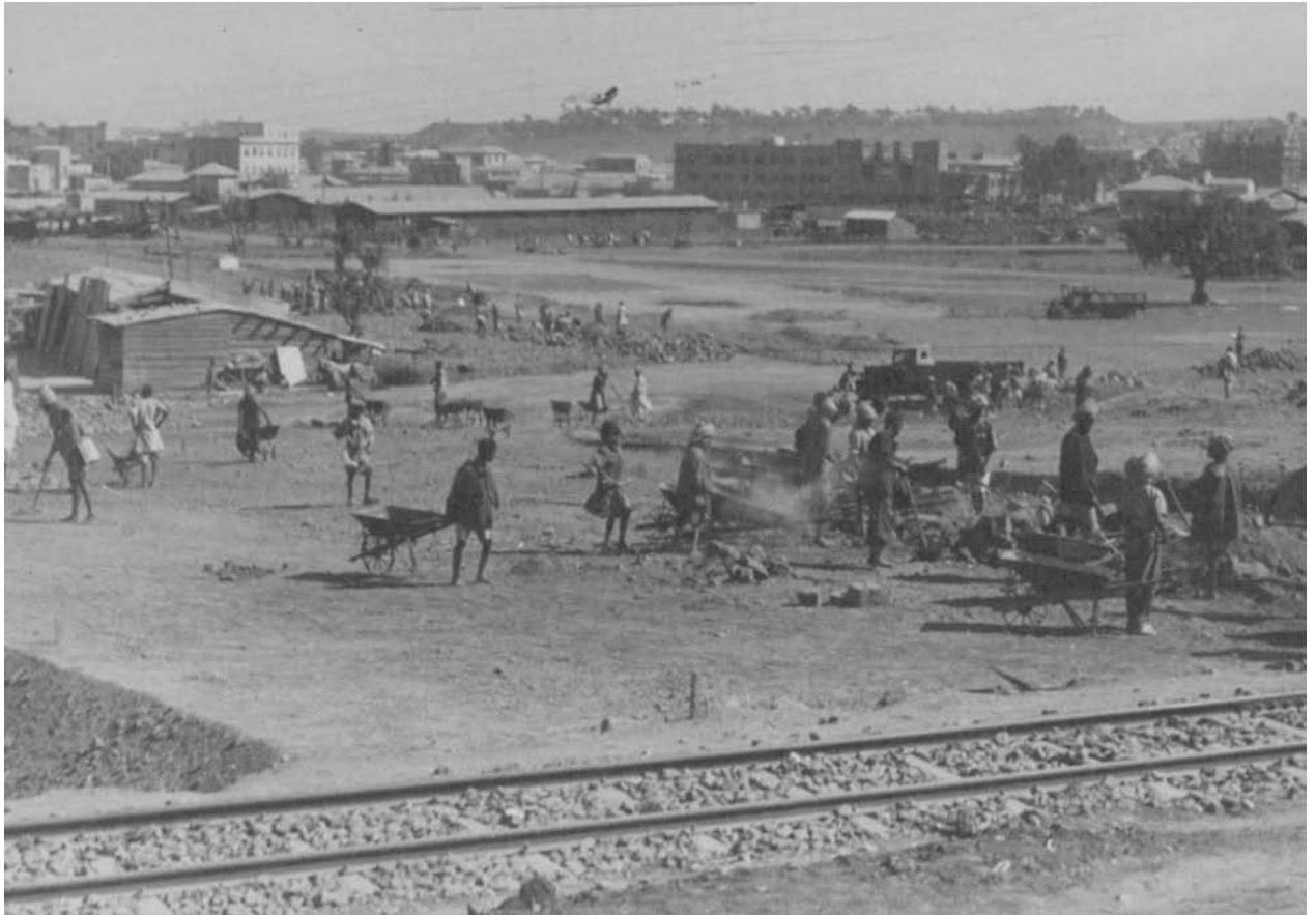
Figs 1.31 - 1.32: Eritrean labourers preparing the terrain in southeast Asmara prior to major urban developments in the mid-1930s. Cinema Impero can be seen under construction in the background. (Below) Eritrean labourers laying major infrastructure under former Viale Mussolini (now Harnet Avenue).
