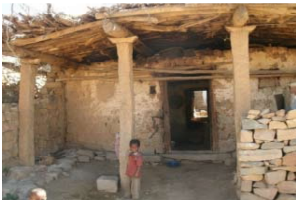
Fig 1.22: Granite columns supporting a roof of tree trunks in a typical old hidmo (over a century old) in Awli-Tsoru village about 35km south of Asmara.
