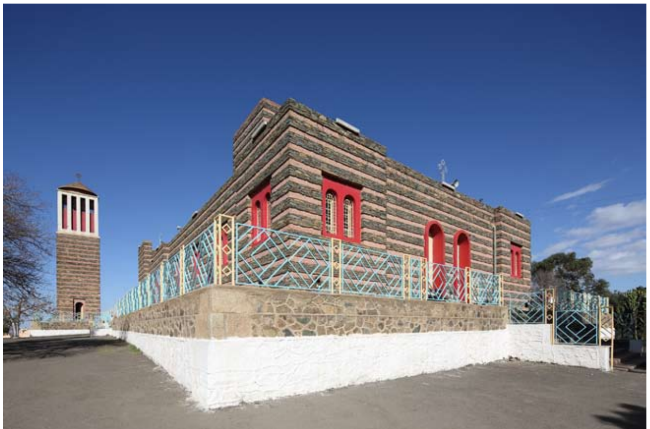
Fig 1.27: Rear of St Mary's Orthodox Cathedral showing the use of basalt and layers of brick, with a foundation of basalt with granite dressings to provide strength at the corners.
