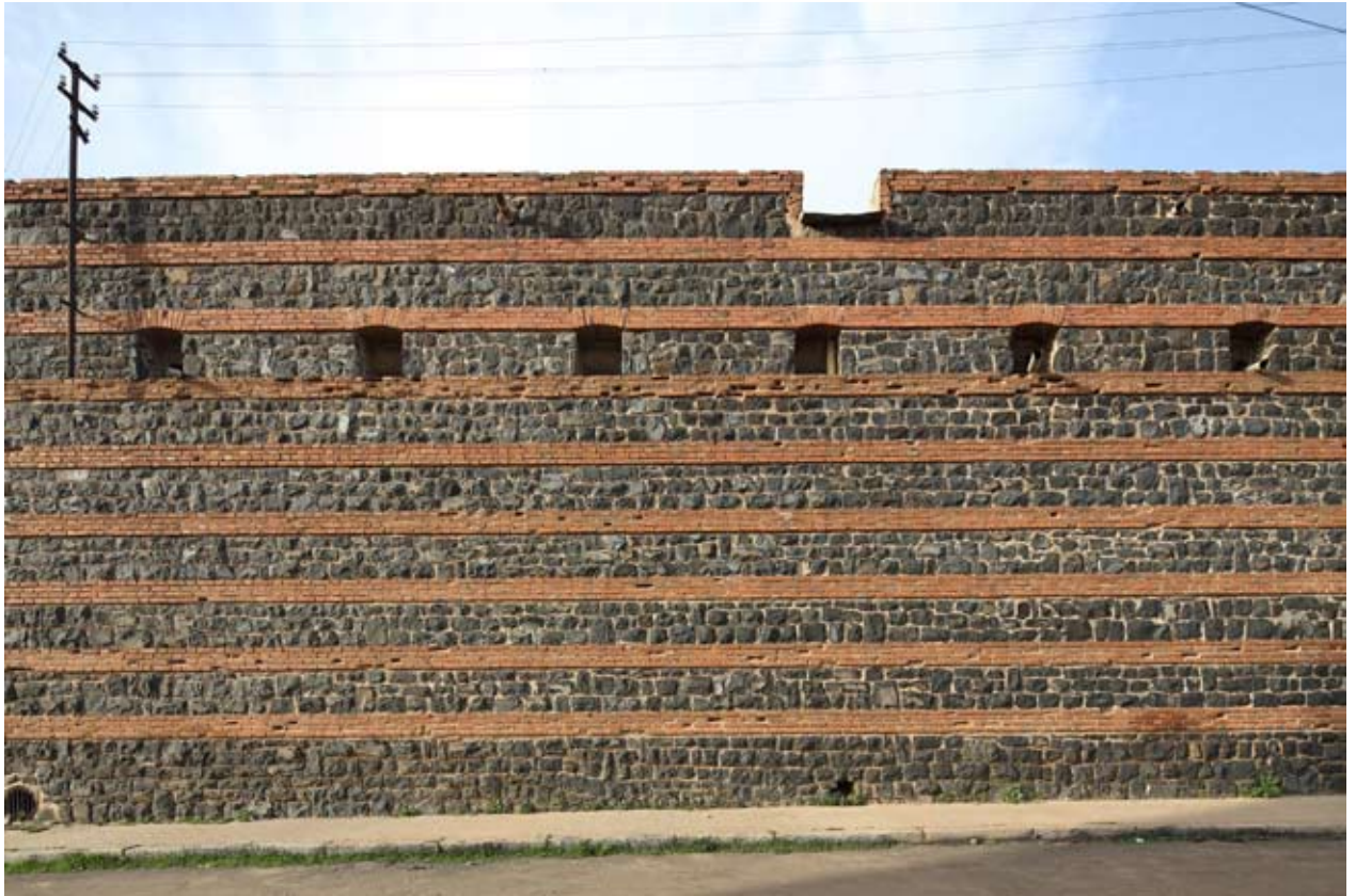
Fig 1.6-1.8: Layers of brick and basalt used in the construction of the massive walls of the Spinelli Store (late 1930s) (above) and (below) similar techniques used in the construction of a Byzantine church from the fourth century AD excavated on the coast of Eritrea in 2014.
