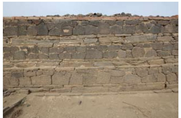
Fig 1.6-1.8: Layers of brick and basalt used in the construction of the massive walls of the Spinelli Store (late 1930s) (above) and (below) similar techniques used in the construction of a Byzantine church from the fourth century AD excavated on the coast of Eritrea in 2014.
