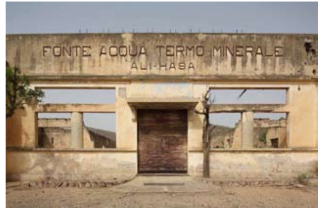
Fig 1.1-1.3: Ruin of a former water processing plant between Asmara and Massawa designed in a modernist style revealing the comparatively conventional building techniques and materials behind the plasterwork to create the desired modernist appearance defined by simple angular and geometric forms and an absence of ornamentation. This example outside the nominated property has been used to illustrate the point because the ruin reveals the underlying structure, which is rare in Asmara owing to the generally good state of conservation.
