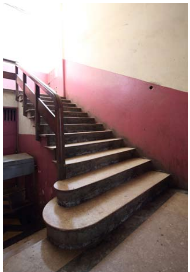
Figs 1.17 - 1.19: (left, bottom) marble polishing machine and (above and below) staircases in 1930s buildings in Asmara with treads and risers of different types of marble.
