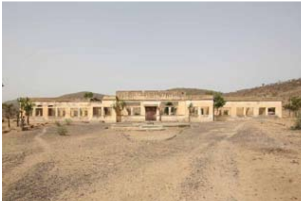
Fig 1.1-1.3: Ruin of a former water processing plant between Asmara and Massawa designed in a modernist style revealing the comparatively conventional building techniques and materials behind the plasterwork to create the desired modernist appearance defined by simple angular and geometric forms and an absence of ornamentation. This example outside the nominated property has been used to illustrate the point because the ruin reveals the underlying structure, which is rare in Asmara owing to the generally good state of conservation.
