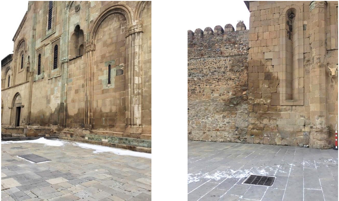
Fig.1 Water track on the southern wall of the Cathedral and the main gate of complex.
