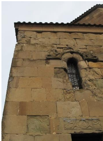
Fig.6 Stone deterioration process on the major church and on the remains of walls
