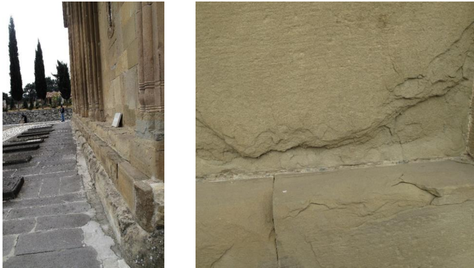
Fig.9 Stone deterioration on the walls of the main church
