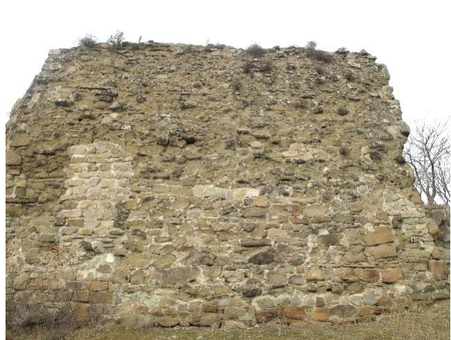
Fig.6 Stone deterioration process on the major church and on the remains of walls
