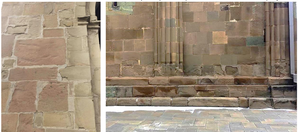
Fig.2 Stone deterioration examples on the walls of cathedral
