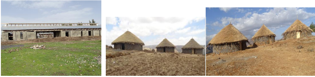
Fig. 8: (A) progress of the Primary school and (B) community lodges; Source: AWF (2016)
