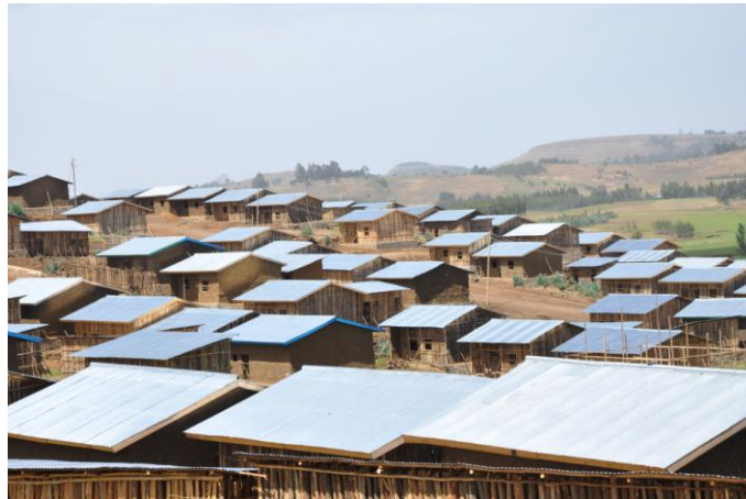
Fig.2: Houses Constructed by Gich community members at Debarik town; Source: LISNMP-ADC (2016)
