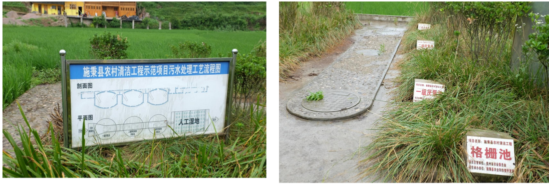
Fig 17 Cleaning project and sewage treating pool in villages
