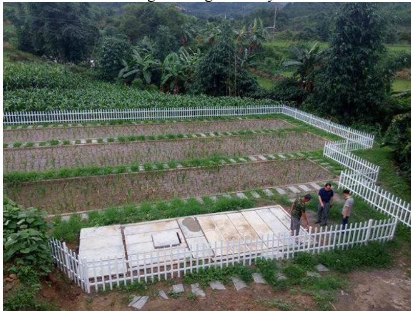
Fig 11 Sewage treatment pool in Libo Karst
