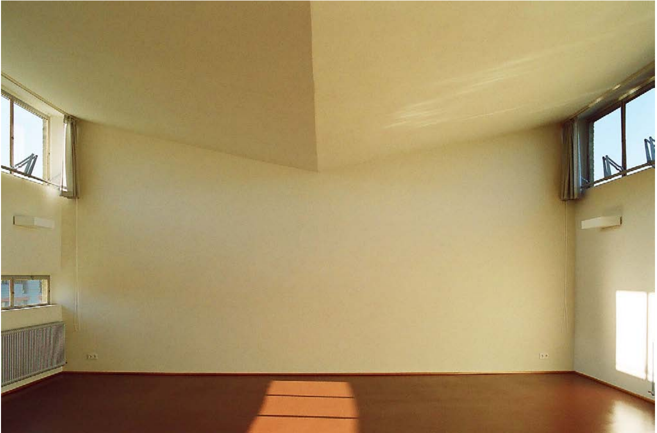
Fig. 39: Seminar room with side ribbon windows and "butterfly ceiling" for optimal natural lighting, photo 2007, Brenne Architekten
