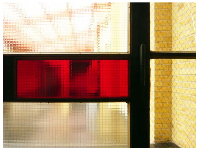
Fig. 2: Coloured reinforced glass on door from the student dormitories to the glass corridor in the ADGB Trade Union School, photo 2009, Brenne Architekten
