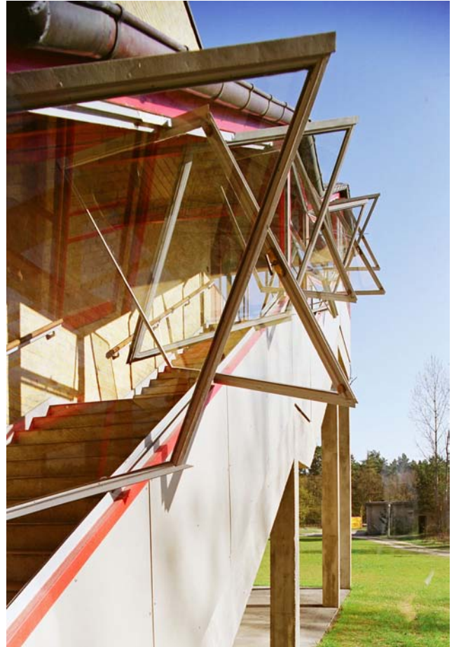
Fig. 36: Detail of new windows in the living rooms reconstructed based on the original models, photo 2007, Brenne Architekten
