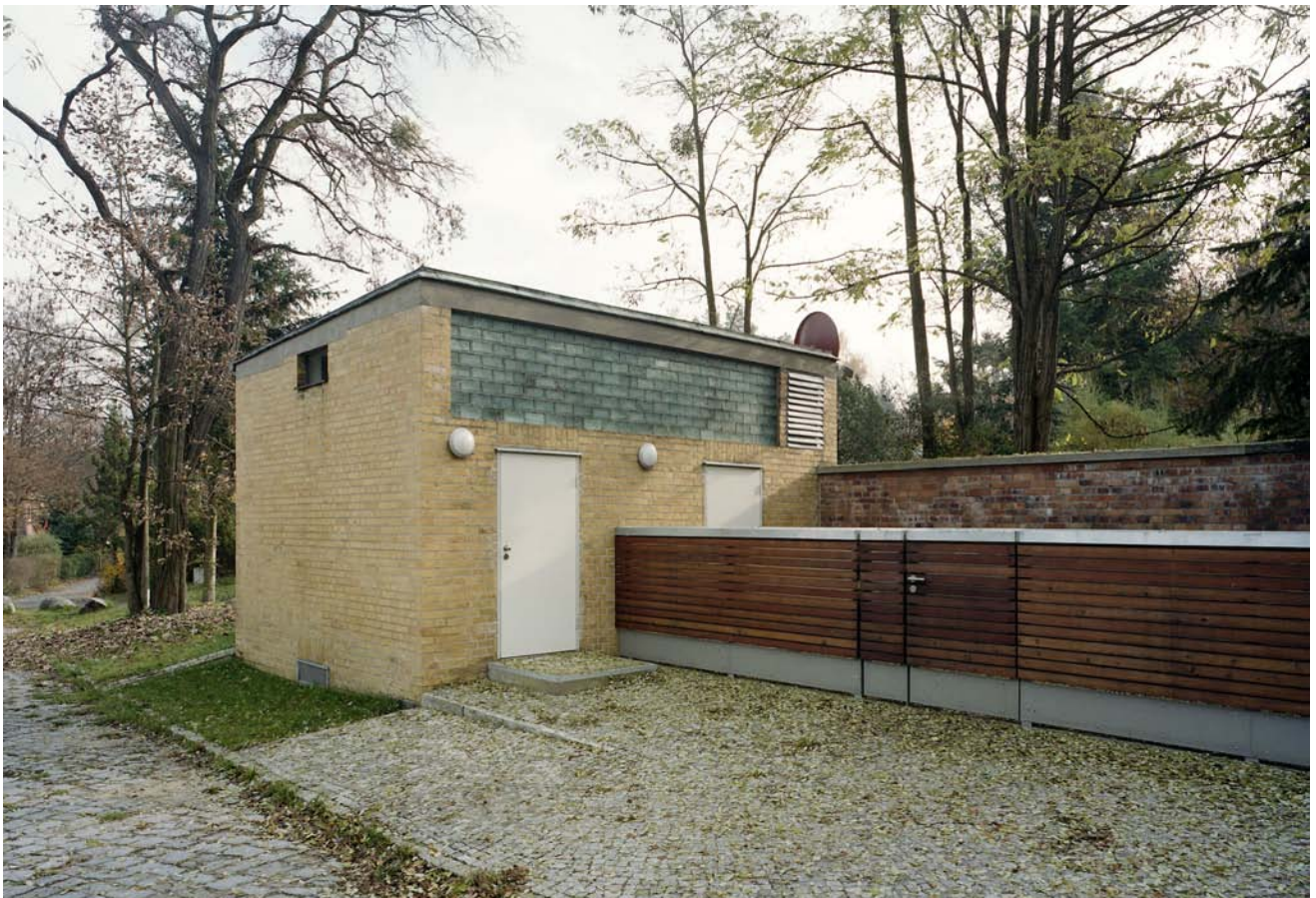
Fig. 43: Original transformer hut with partition for refuse collection area added at a later date, photo 2011, Holger Herschel, Brenne Architekten
