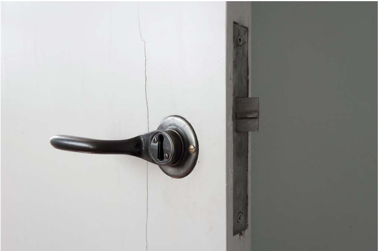
Fig. 20: Original door handle with Odarra lock with integrated keyhole, photo 2012, Bauhaus Dessau Foundation, Sebastian Gündel
