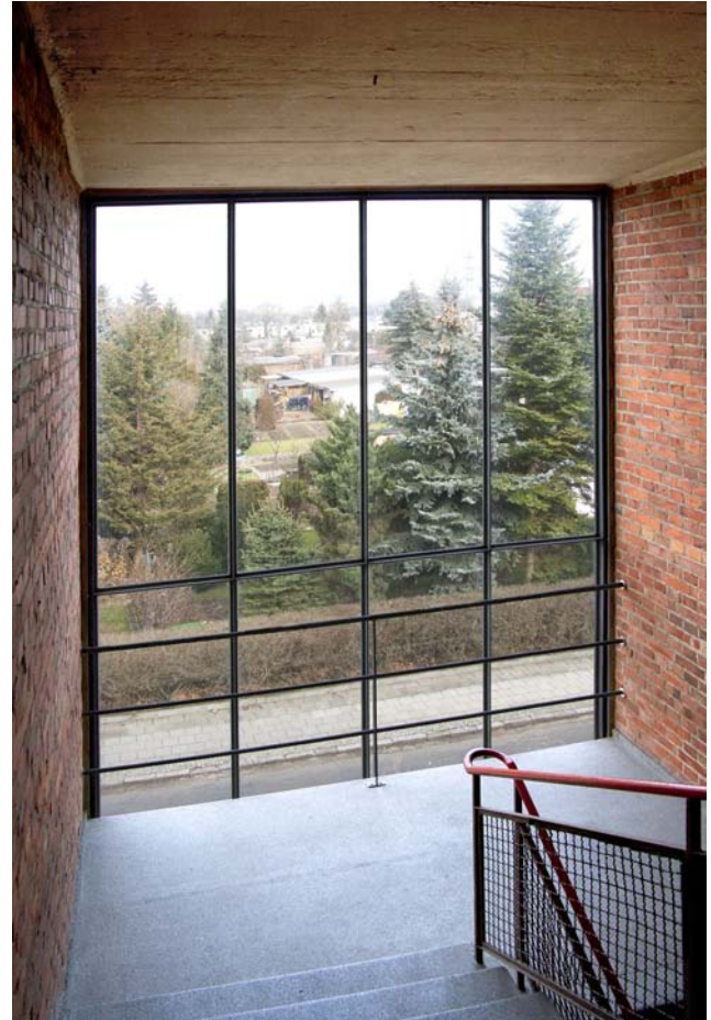
Fig. 11: Stairwell in the House with Balcony Access at Peterholzstraße 40 restored to its original condition with full facade glazing, photo 2012, Bauhaus Dessau Foundation, Yvonne Tenschert
