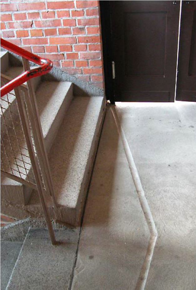
Fig. 10: Drainage channel in stairwell, photo 2004, Bauhaus Dessau Foundation, Bettina Lietz
