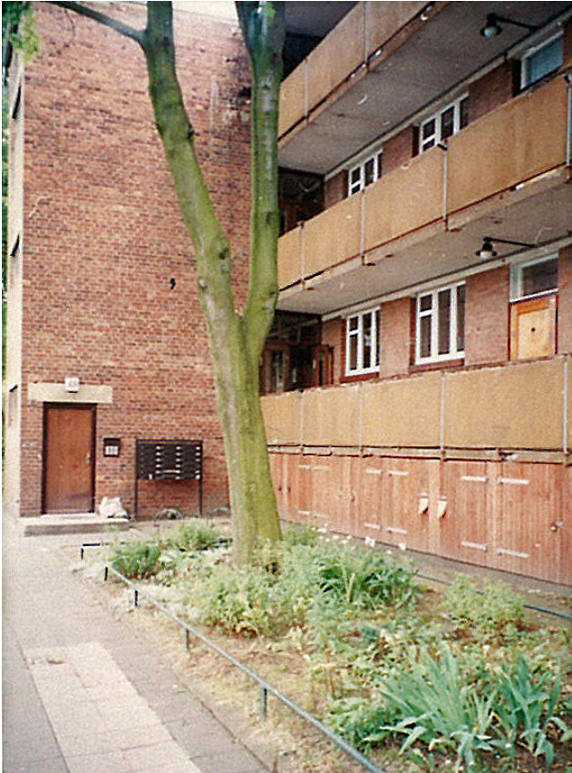
Fig. 59: House with Balcony Access with concrete parapets prior to restoration, photo 1996, Brenne Architekten
