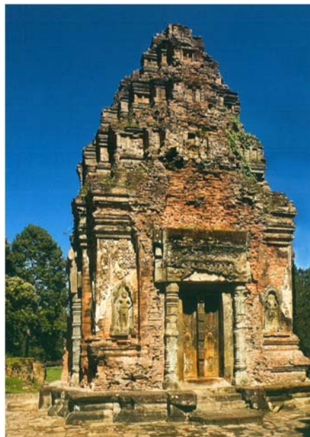
Fig. 3.12 Roluos, Preah Ko, east row, north tower, west façade. The receding storeys are decorated with miniature depictions of towers and supported by interior corbeling, (Brukoff, B. and Jessup, H.I., 2011, p. 34).
