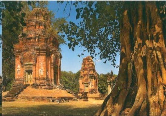
Fig. 3.14 Roluos, Bakong, view of two of the subsidiary towers surrounding the temple. The pediments and guardian Fig.s in arcuated niches flanking the doors are carved from thick stucco and the underlying brick. The collonettes are cylindrical, as in seventh-century temples..., (Brukoff, B. and Jessup, H.I., 2011, p. 44).
