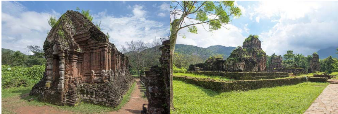
Fig. 3.19 & 3.20 The temples at My Son are made of a reddish brick. Decorative carvings have been cut directly into the bricks.
