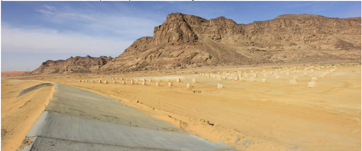
Work underway to frame and mask the rain water divisionary dam/water barrier with typical low desert vegetation to preserve the long term visual integrity of the site
