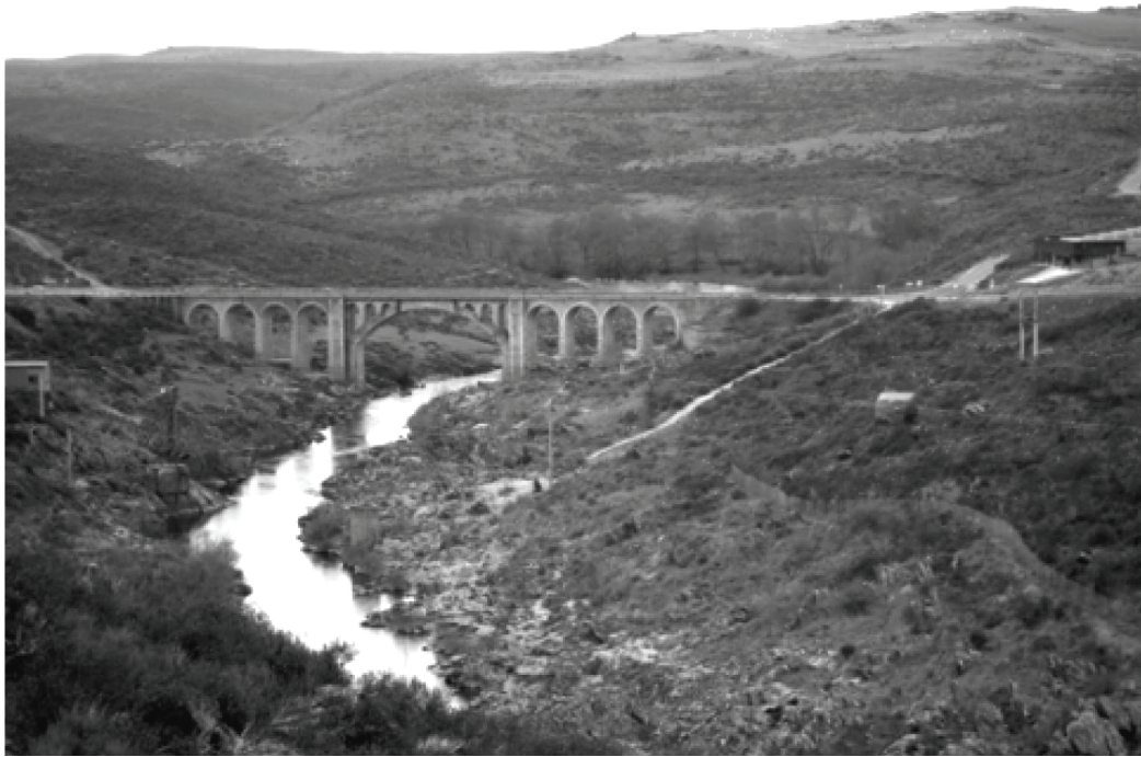
General view of the nominated property
