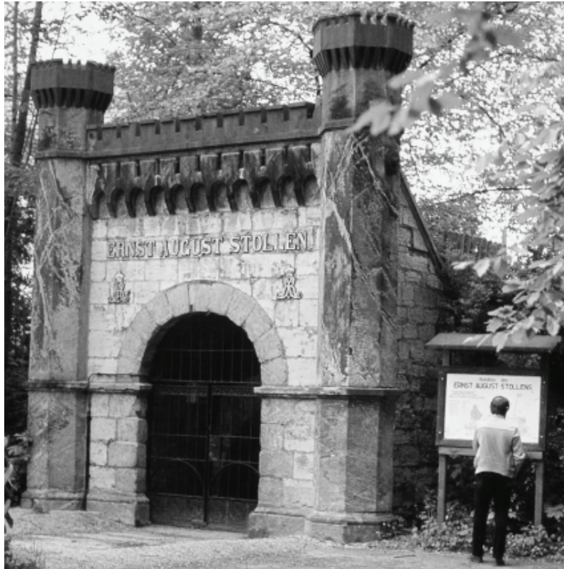
Ernst-August-Stollen underground drainage gallery
