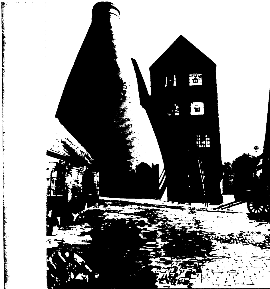
11. Courtyard, China Works at Coalport
