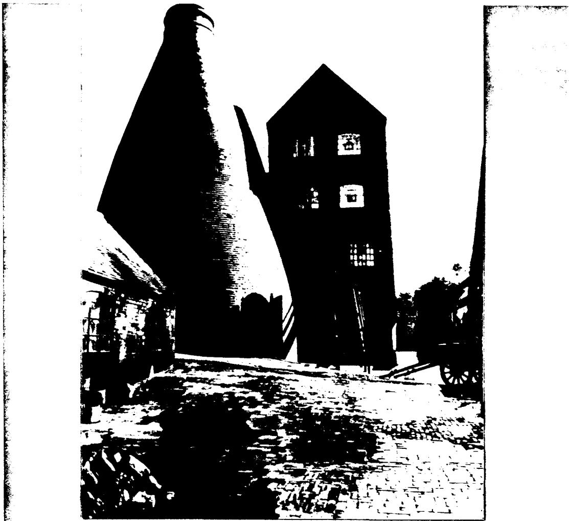
11. Courtyard, China Works at Coalport
