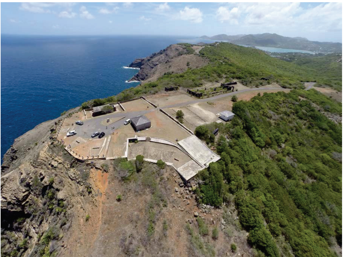
Aerial view of Blockhouse complex with Cistern, Gun Platforms and Powder Magazine
